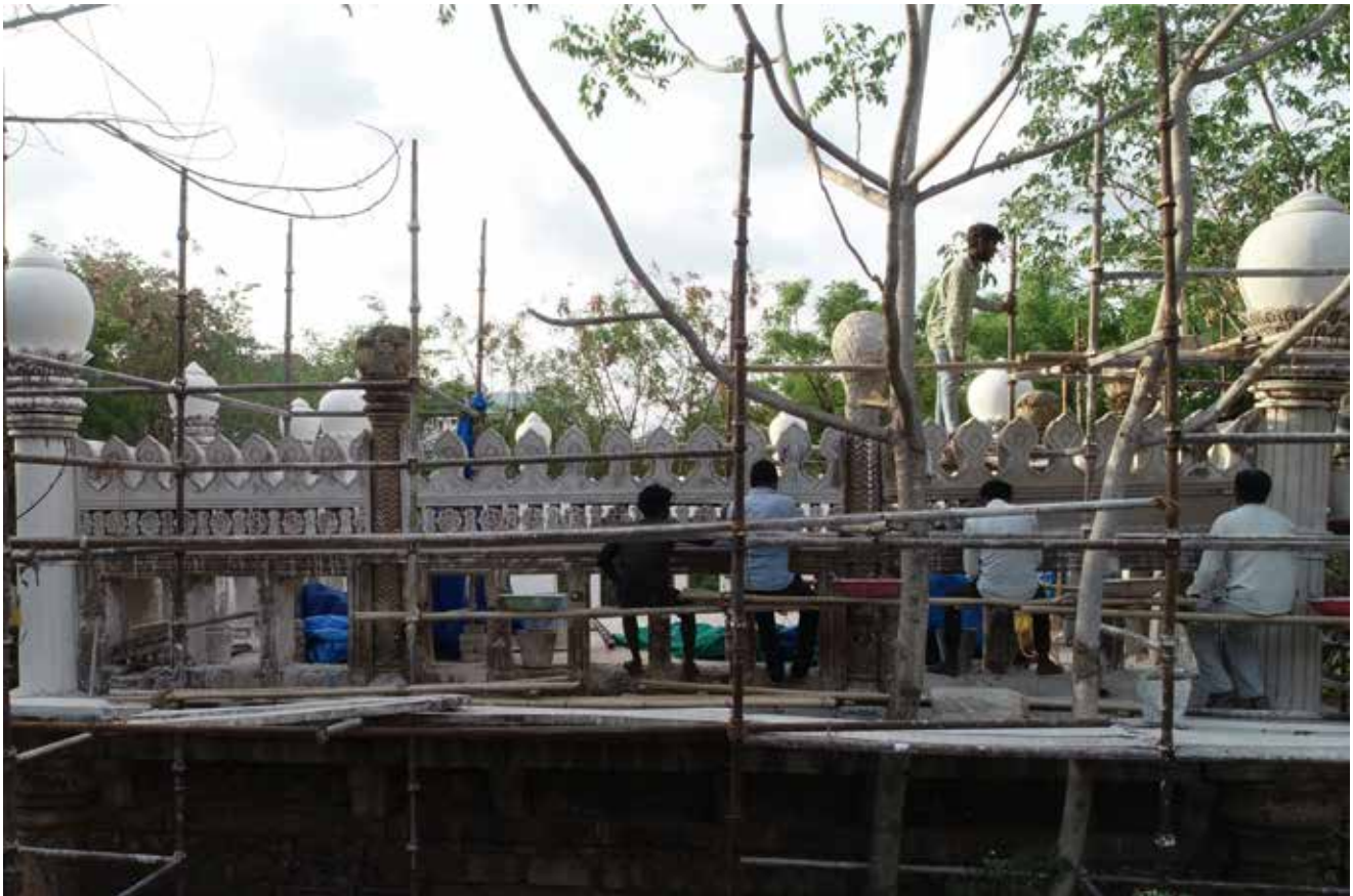
Damaged minarets, missing merlons, and decorative lime stucco details on the parapet being restored carefully by skilled craftsmen
