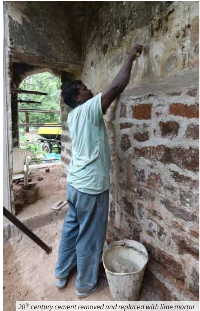
Lime repairs on the main facade of the mausoleum
