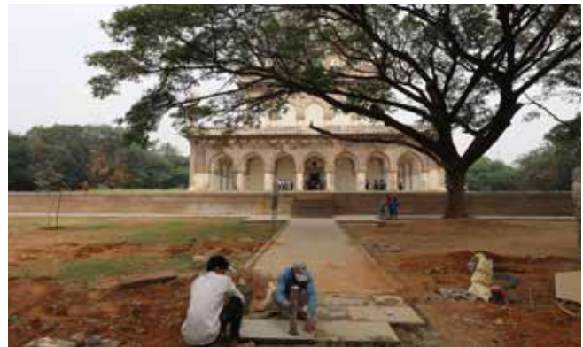
(Left) Installation of tandur pathway east of Taramati and Premamatis mausoleum (Right) Laying of pathway south of Abdullah Qutb Shahs mausoleum
