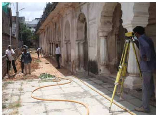
Flooring around the monuments was relaid in an appropriate slope based on the workings and slope of the historic drainage system
