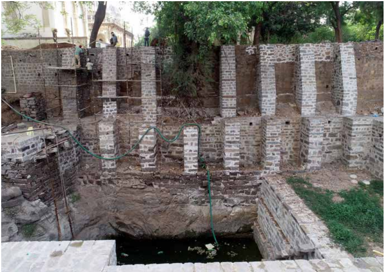
Construction of counterforts by skilled stone artisans
