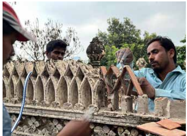
(Clockwise from Left) Reinstating lattice screen around the graves; Reconstruction of parapet by mastercraftsman; Based on existing evidence, interlocking jaali work reconstructed using terracotta pieces; Broken or missing minarets are being restored
