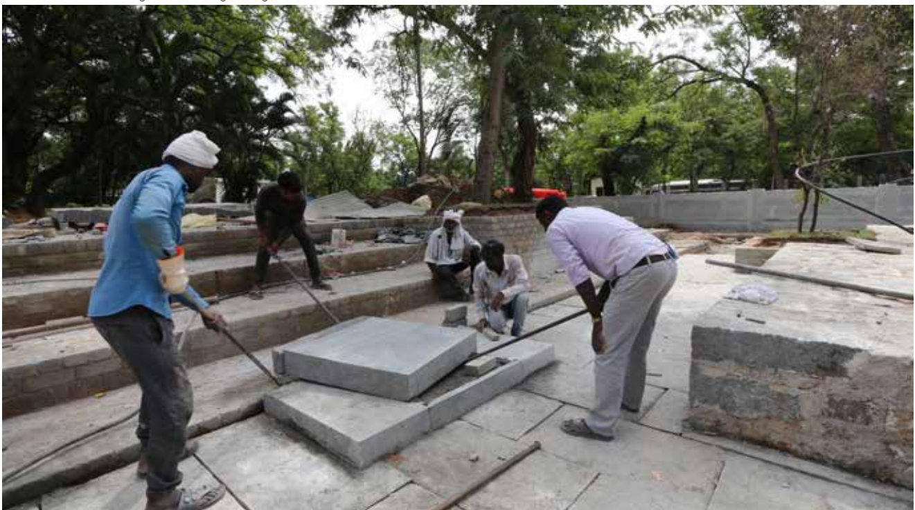
Skilled artisans installing stone seating at Bagh Baoli
