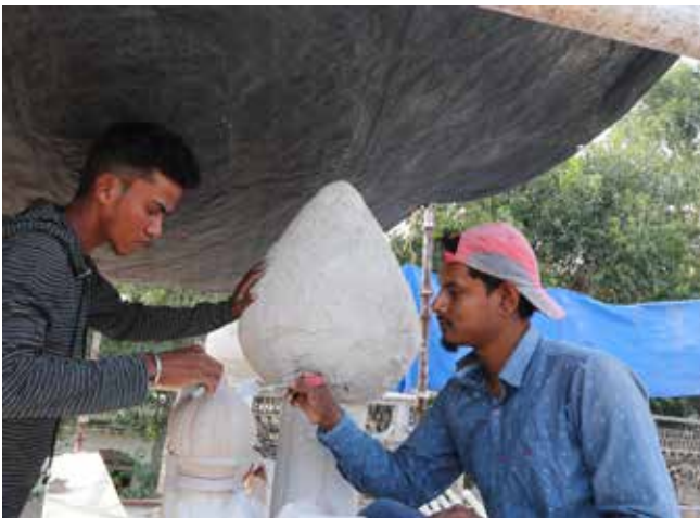
(Clockwise from Left) Reinstating lattice screen around the graves; Reconstruction of parapet by mastercraftsman; Based on existing evidence, interlocking jaali work reconstructed using terracotta pieces; Broken or missing minarets are being restored
