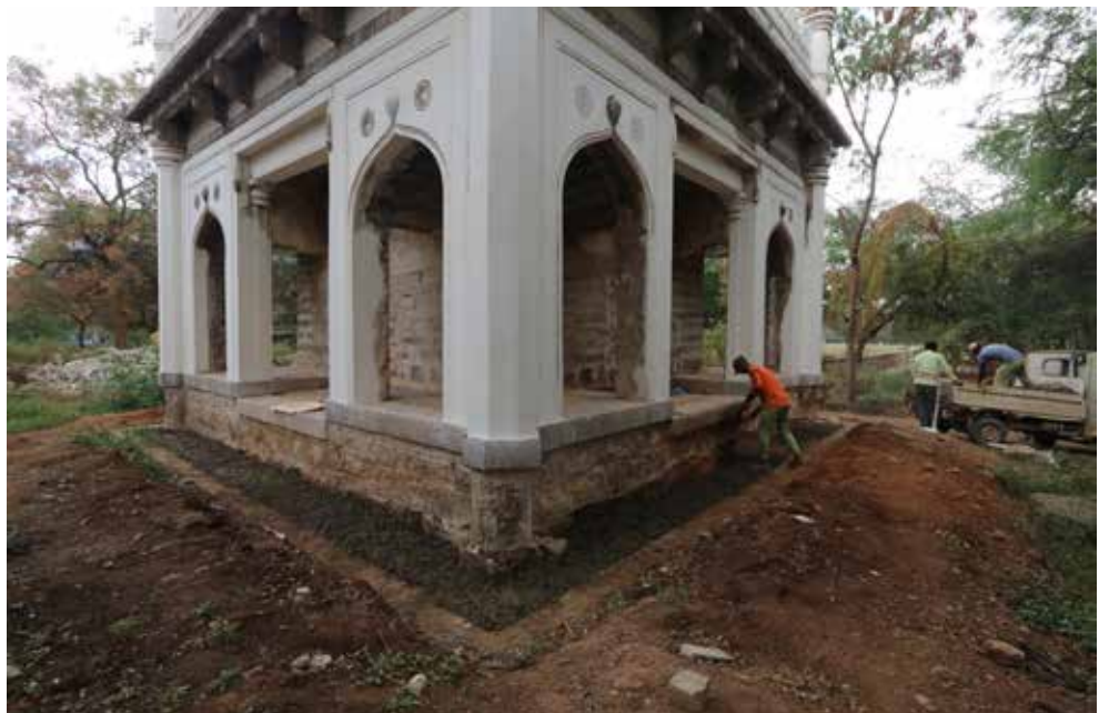
(Top) Scientific clearance to determine the original plinth levels of the monument; (Bottom) Base work has been completed for the laying of plinth protection around the monument
