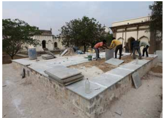
(Left) Precise placement of stone lintels on the eastern entrance; (Right) Laying of stone flooring on the upper platform in an appropriate slope
