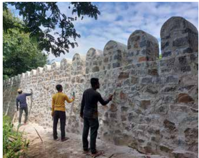
(Top) Craftsmen used the original evidence for reconstruction of battlements; (Bottom) Lime repointing of the wall after removal of cement layers
