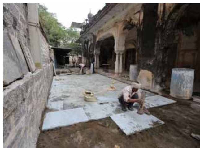
Flooring around the monuments was relaid in an appropriate slope based on the workings and slope of the historic drainage system
