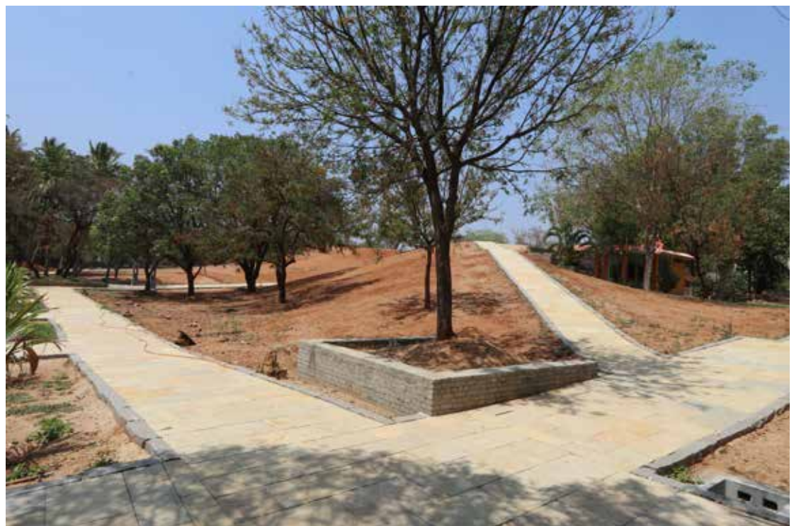
(Top) Retaining wall constructed along the ecological area to slow down surface water movement; (Bottom) Toe walls built around trees at the Mound in Deccan Park
