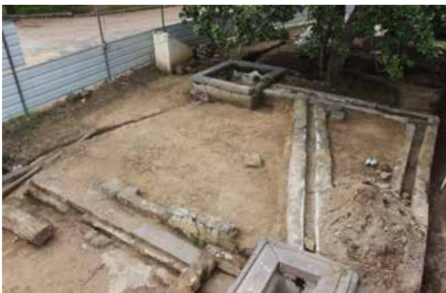
Restoration of the water channels and cisterns to their original slope and profile
