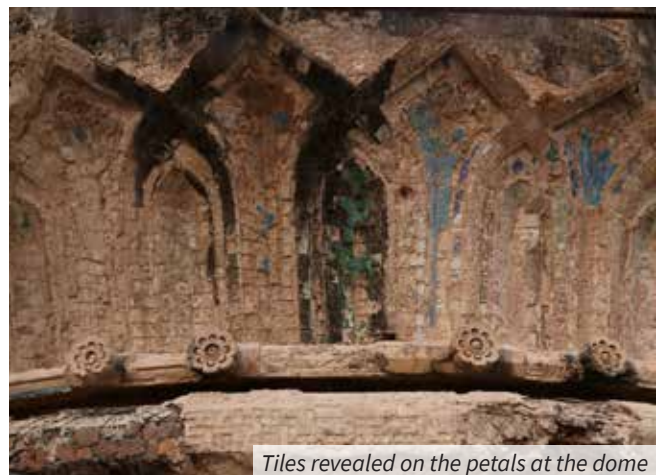
Investigations on the dome to reveal tile layer
