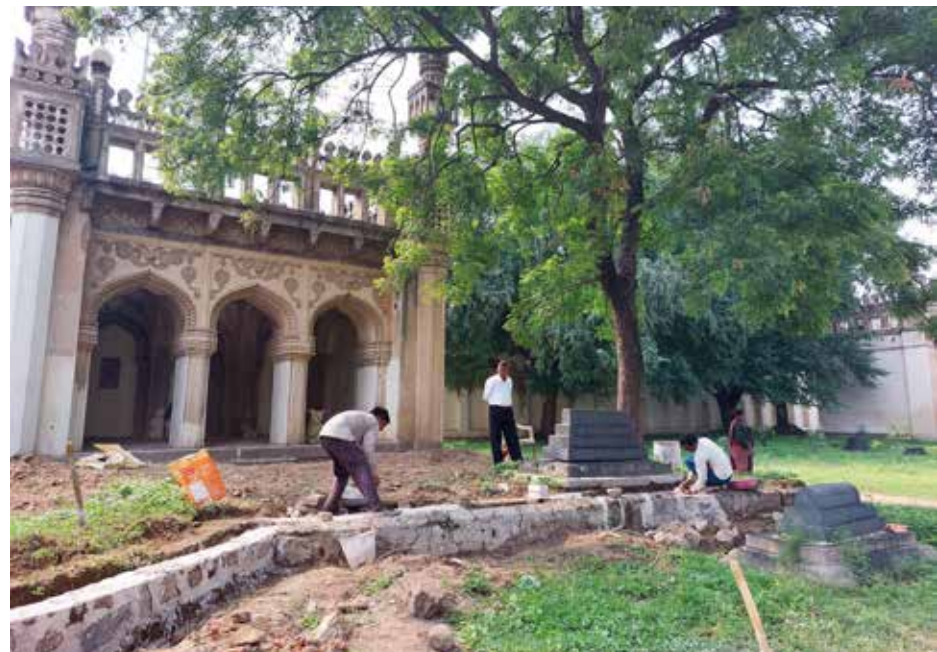
(Above) Skilled craftsmen restore traditional lime plaster on the eastern plinth wall, replacing the 20 th -century cement plaster at Hayat Baksh Begum's mausoleum; (Below) Consolidation of water channels at Funerary Mosque No. 8*
