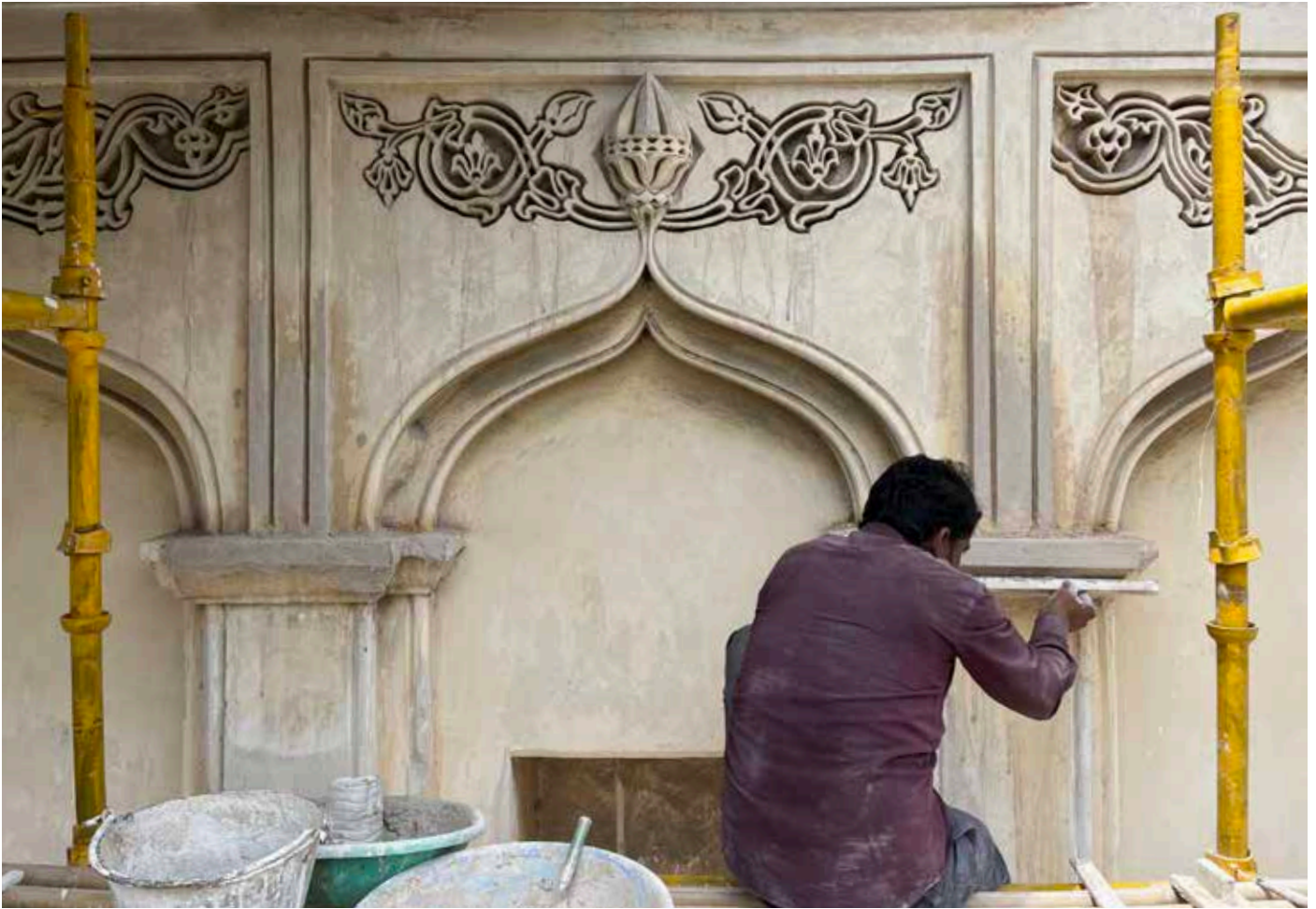
Damaged capital bands repaired using traditional lime plaster at the middle level facade
