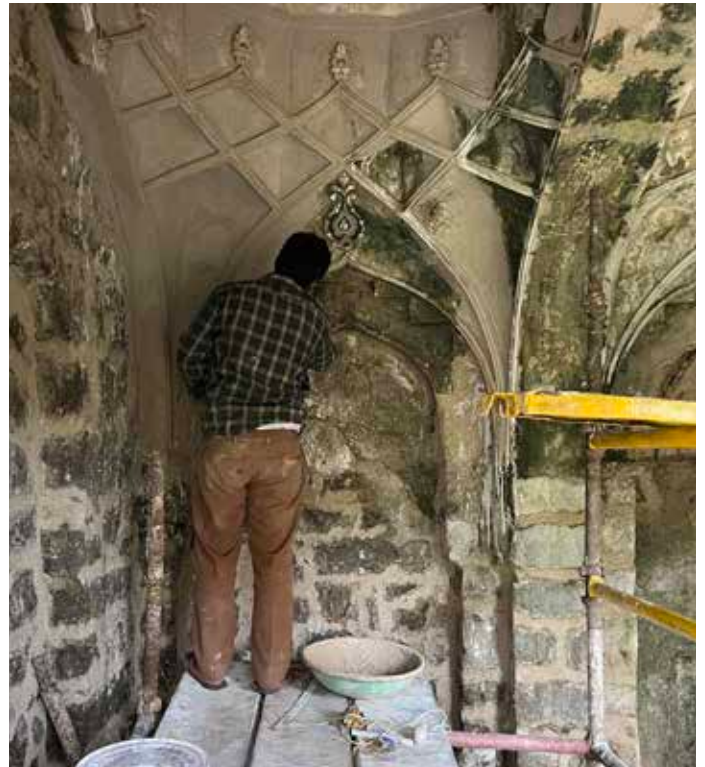
The internal wall surfaces were restored using traditional lime mortar
