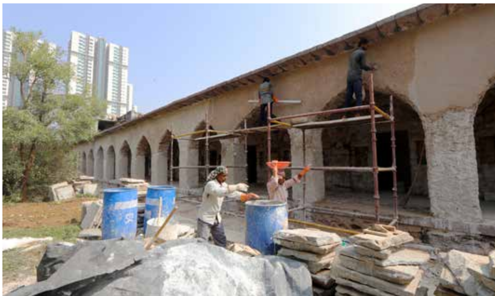
Replastering the arches of the facade with traditional lime plaster after removing the 20 th century cement plaster
