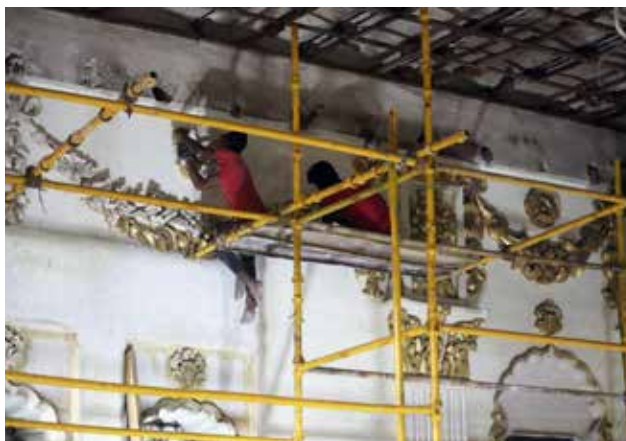
'later added golden enamel paint obscuring the original stucco patterns has been carefully cleaned to reveal the original details.
