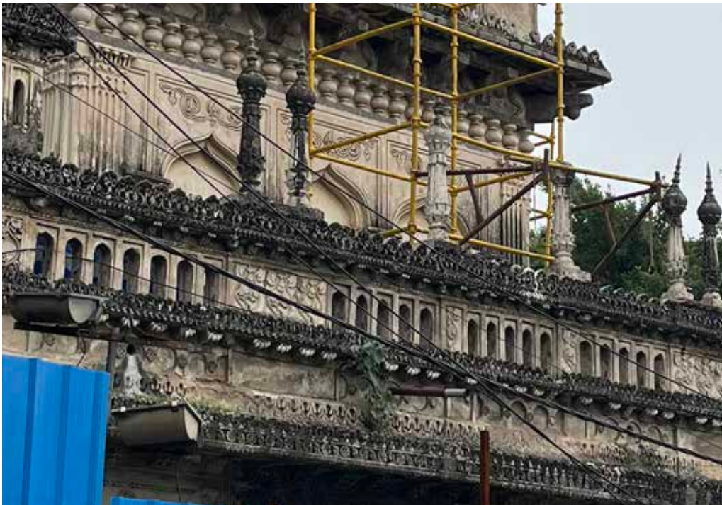
During previous repairs, the original decorative lime stucco panels were replaced with pre-cast cement motifs
