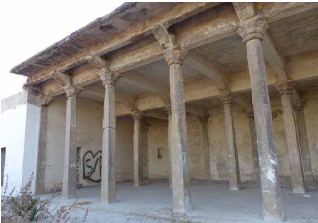
The interior of the stable before conservation, featuring high hand-chiseled granite stone columns
