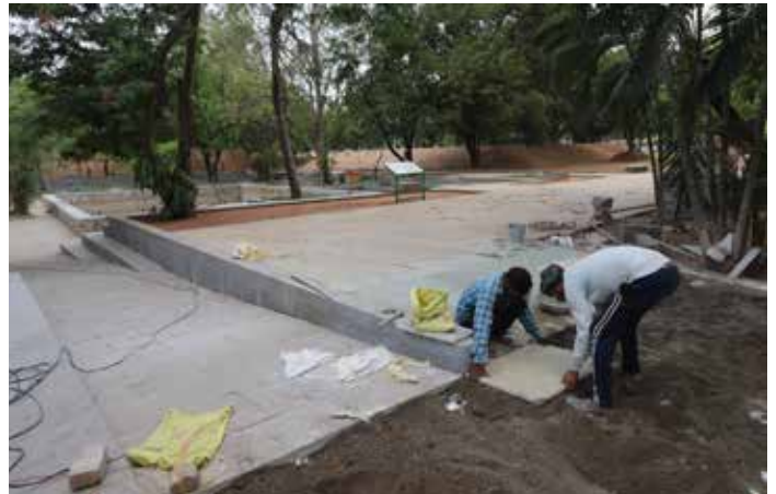
Laying tandur stones at the ramp was for universal access
