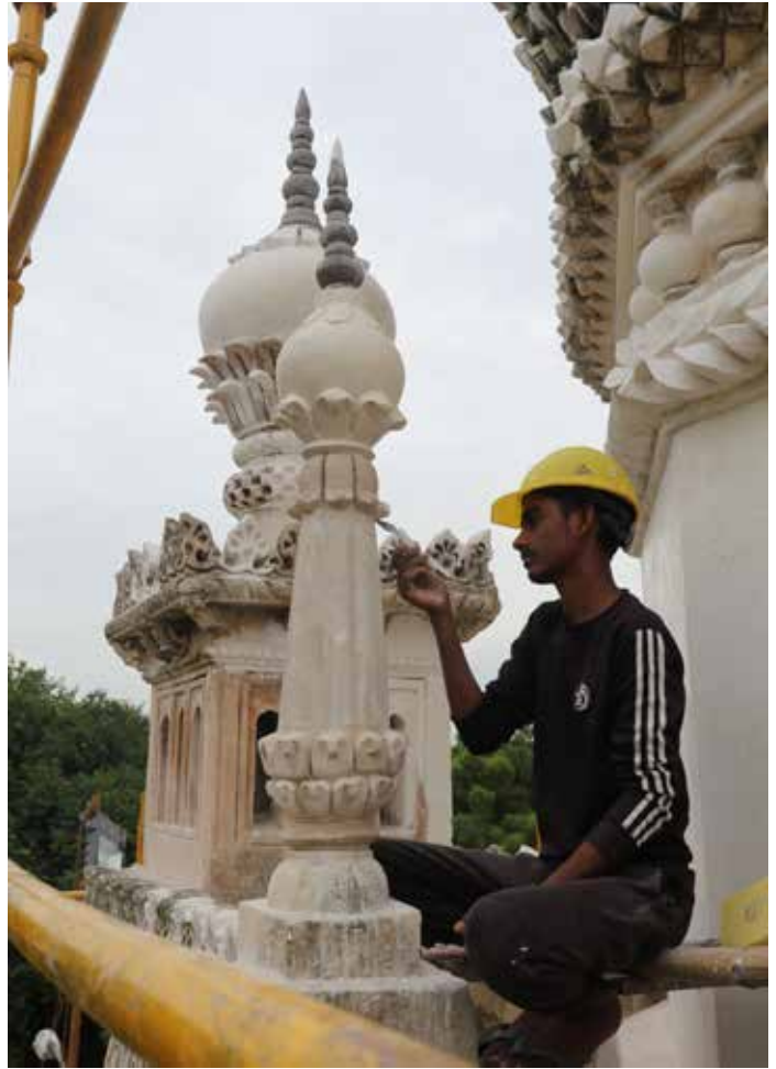
The dilapidated minarets were restored by repairing broken elements and recreating missing details
