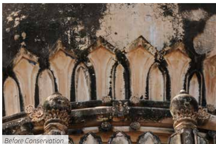
Original tiles revealed on removal of 20 th century cement
