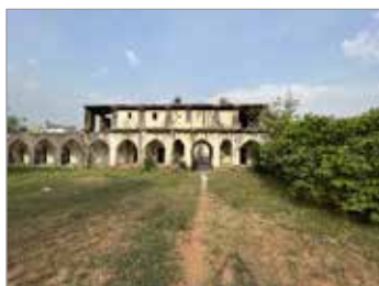
West Elevation - 20th century cement plaster, uneven arch profiles Black Crust, flaking of plaster layer , deteriorated plaster layer, water seepage, missing lime stucco details, missing chajja stone, missing and damaged parapet
