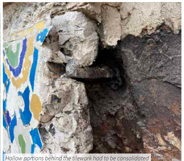
Damaged portion of the facade, the black basalt edging had fallen and there was a risk of tilework falling
