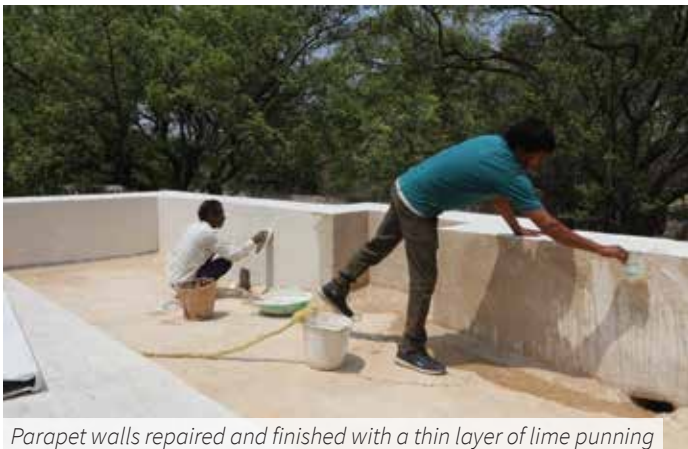
Traditional lime concrete laid on terrace replacing the 20 th century cement
