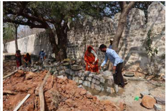
(Clockwise from left-top) Reconstruction(matching the original) of missing masonry walls and arches using formwork; Replastering the masonry walls and arches with traditional lime mortar matching the original details of the enclosure wall; Plinth protection using stone masonry walls along the northern enclosure wall; Finishing of the plinth protection with laying of 30 mm tandoor stone along a portion of the western enclosure wall
