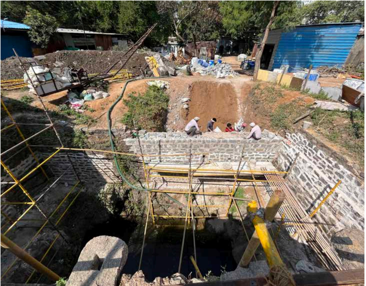
The collapsed western wall of the baoli was rebuilt to match the original offsets, and weepholes at intermediate levels were provided to facilitate drainage
