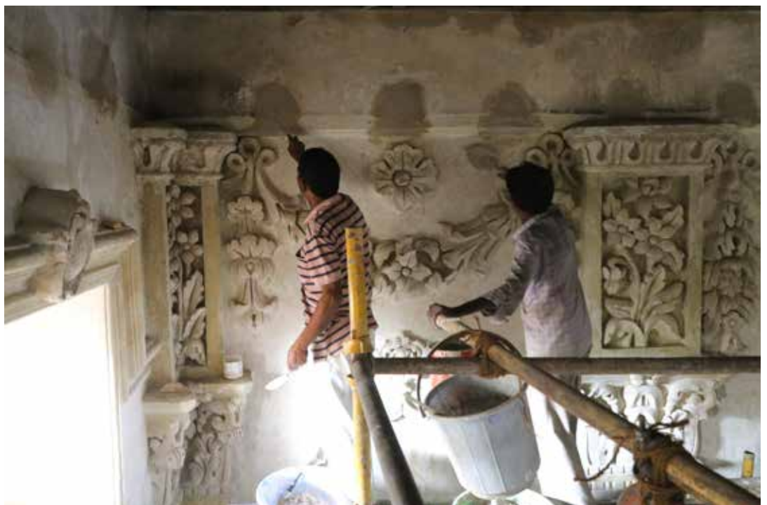
(Top) Exposed jack arches have been carefully plastered with traditional lime mortar for long-term preservation; (Bottom) Damage ornamental lime stucco details restored by master craftspeople
