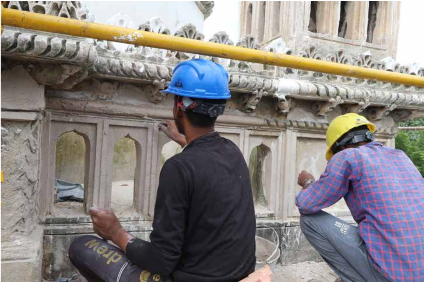
Broken portions of the parapet were repaired and restored using lime mortar
