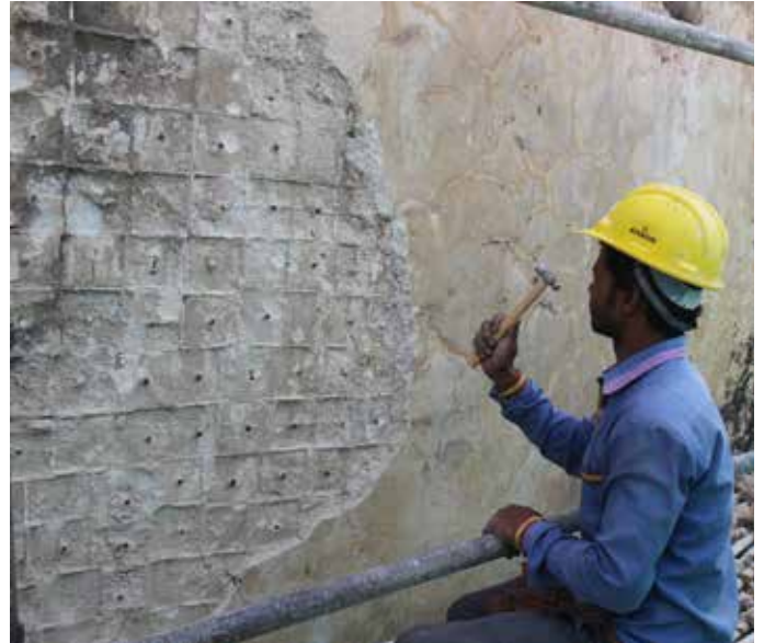
20 th century cement layers were carefully removed, revealing original tiles held in place with iron nails. Iron nails were historically used to secure tiles along the dome's curve
