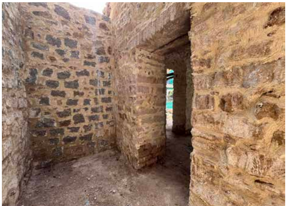
Partly collapsed stone masonry wall is reconstructed to restore the original layout of the building
