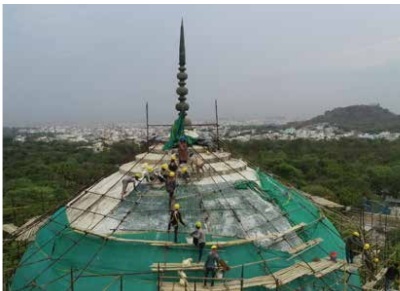
Skilled craftspeople installed over 80,000 tiles, covering 850 square meters of the dome surface
