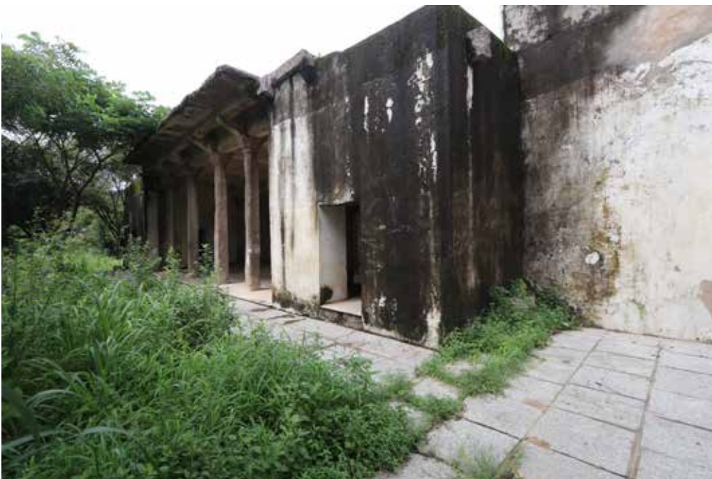
Algae deposition from water seepage has severely damaged the external facade of the stable
