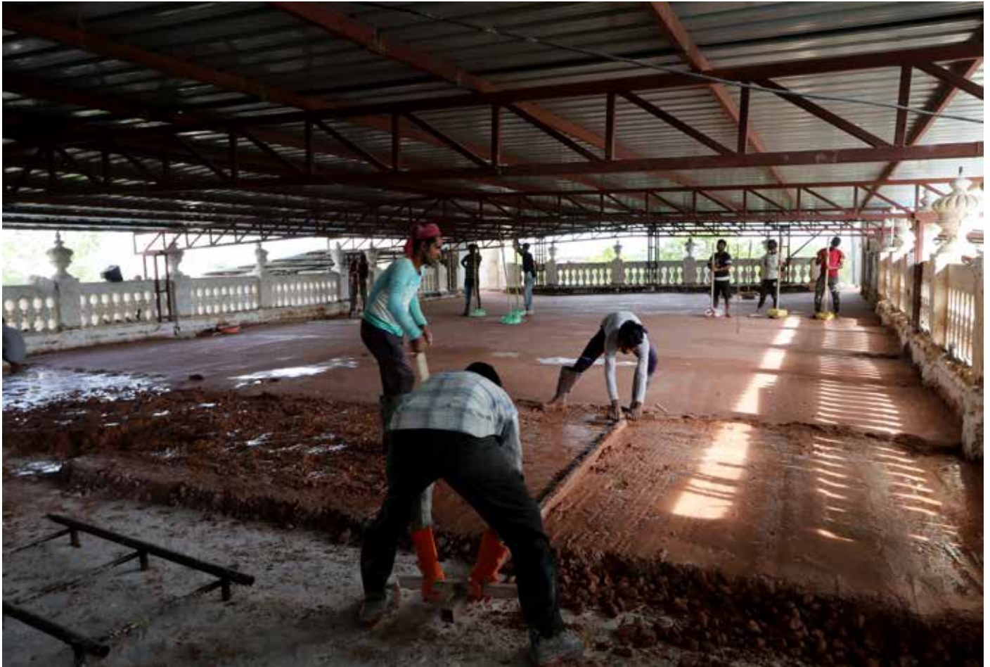
Laying lime brick jelly concrete on the main hall terrace to adequate slope, after dismantling of later added cement concrete
