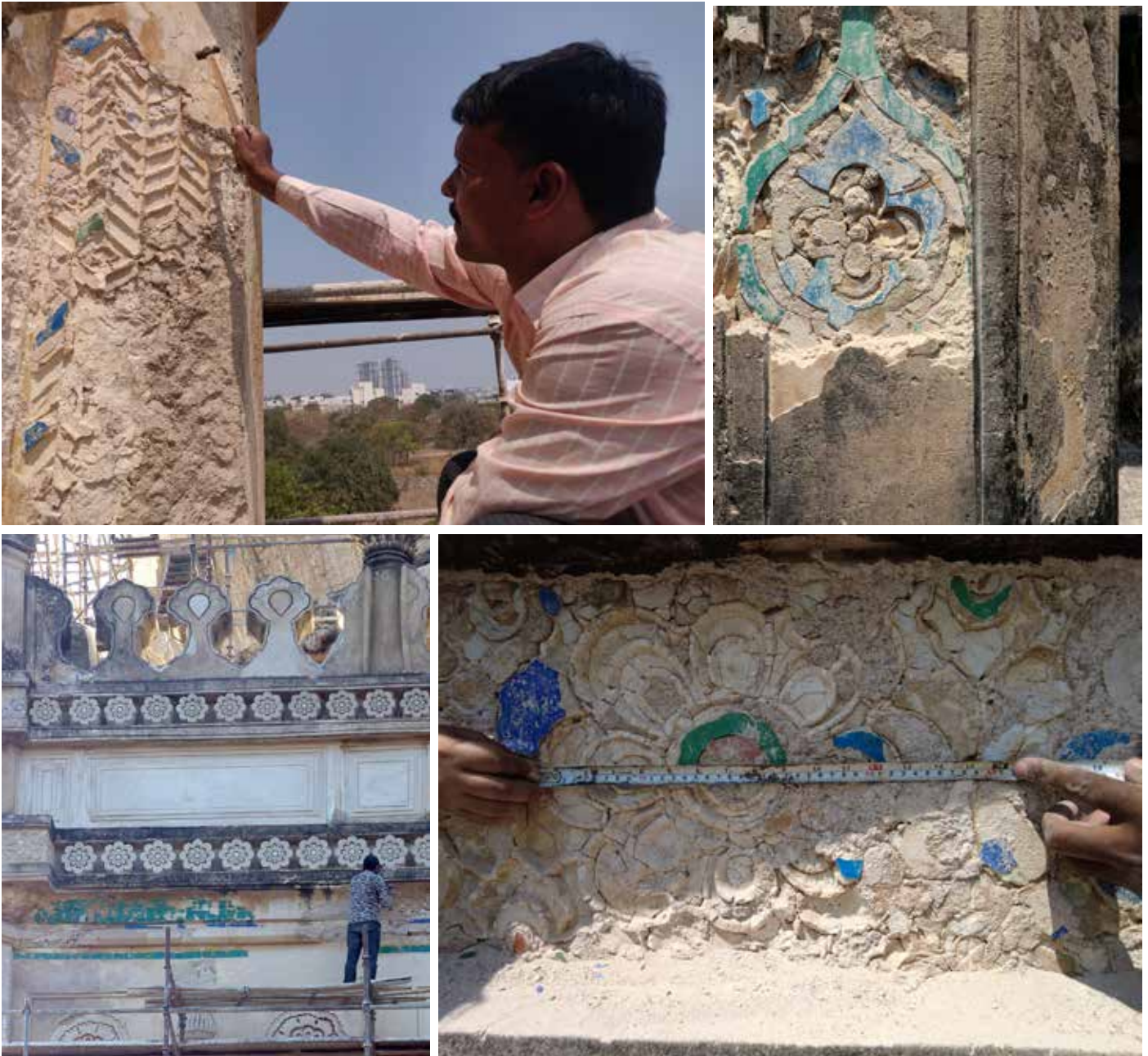
Remnants of original glazed tiles and tile patterns revealed on various portions of the mausoleum, including the facade and corner columns
