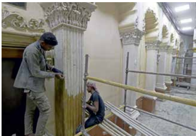
'later added golden enamel paint obscuring the original stucco patterns has been carefully cleaned to reveal the original details.
