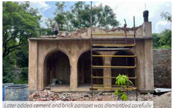
Later added cement and brick parapet was dismantled carefully
