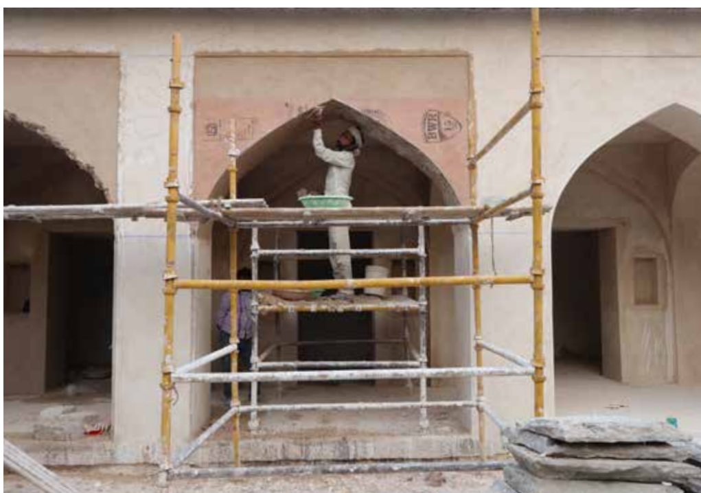
Reinstating the arched facade of the Sarai to ensure uniformity in level, size, and shape
