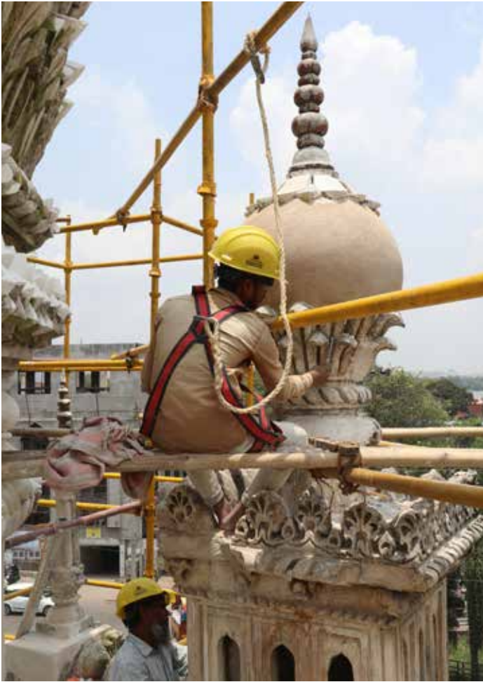
The dilapidated minarets were restored by repairing broken elements and recreating missing details
