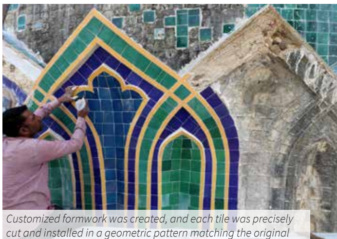
Original tiles revealed on removal of 20 th century cement
