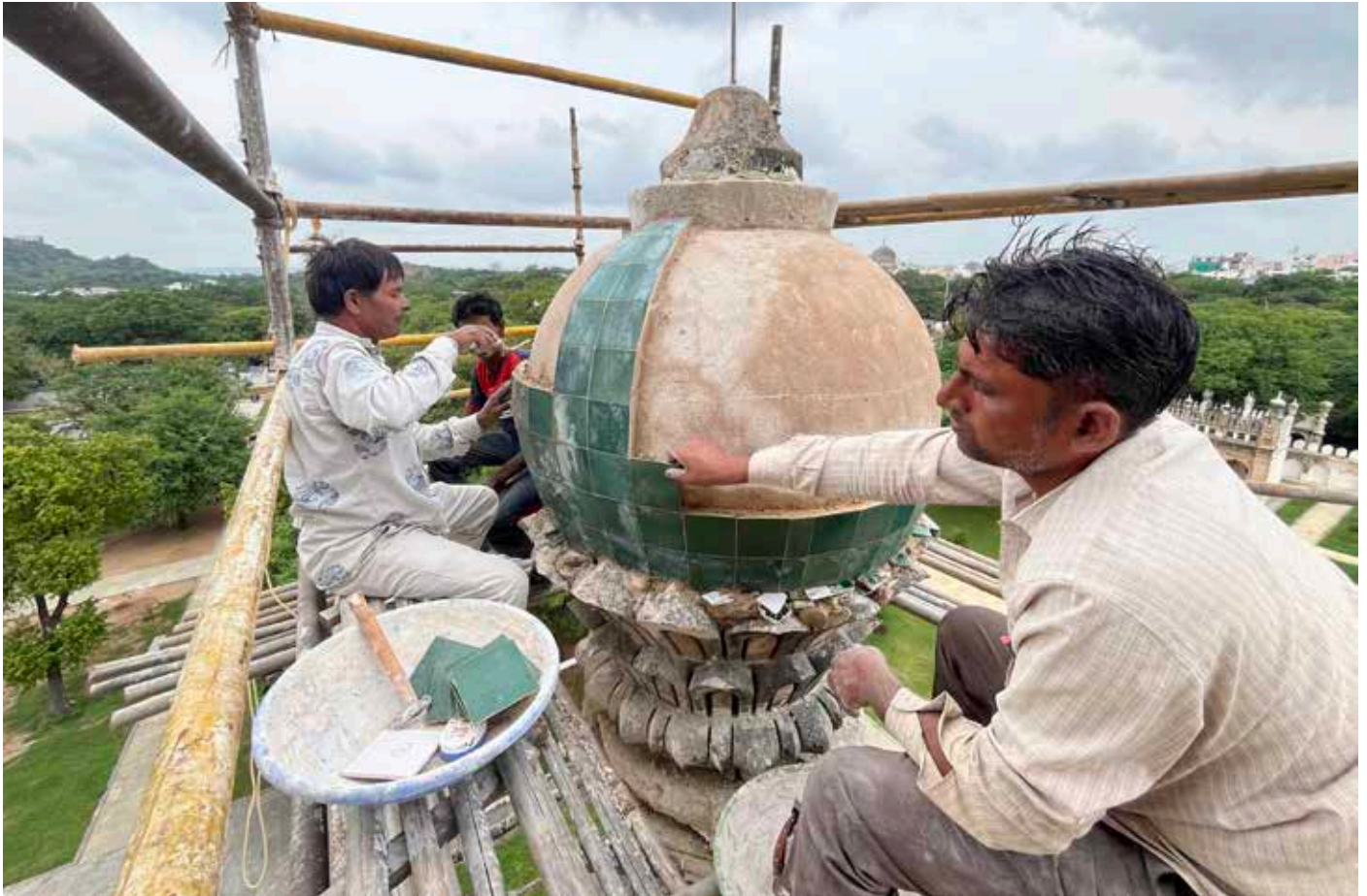
Tiles were installed by master craftspeople after consolidating the minaret bulbs with traditional lime mortar
