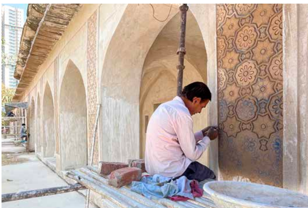
Taking cue from the existing ornamentation on site, missing lime stucco work was restored by skilled craftspeople
