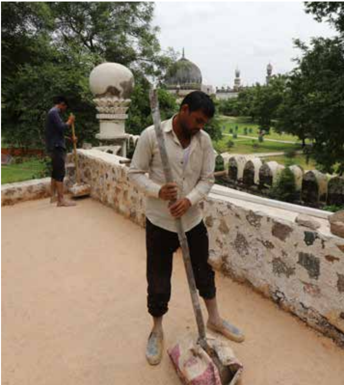
Compaction of traditional lime concrete laid on the repaired terrace
