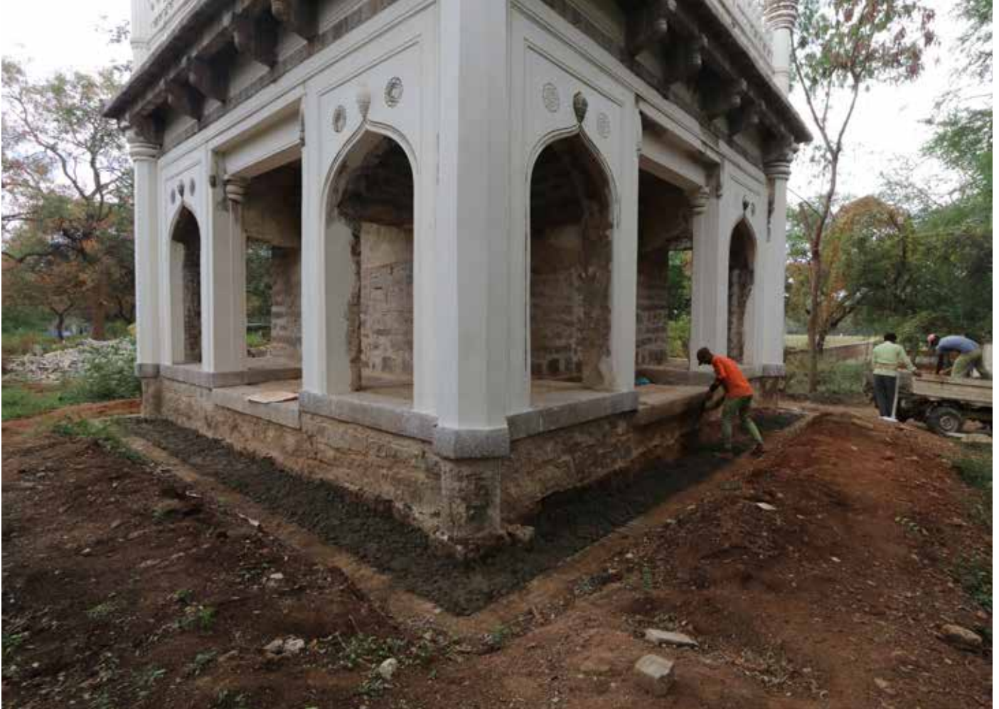
Base work for the laying of plinth protection around the monument
