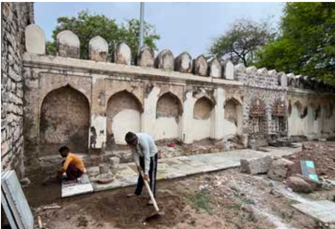
(Clockwise from left-top) Reconstruction(matching the original) of missing masonry walls and arches using formwork; Replastering the masonry walls and arches with traditional lime mortar matching the original details of the enclosure wall; Plinth protection using stone masonry walls along the northern enclosure wall; Finishing of the plinth protection with laying of 30 mm tandoor stone along a portion of the western enclosure wall
