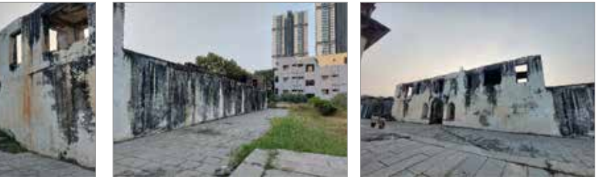
- Black Crust, flaking of platelayer , deteriorated plaster layer, water seepage
