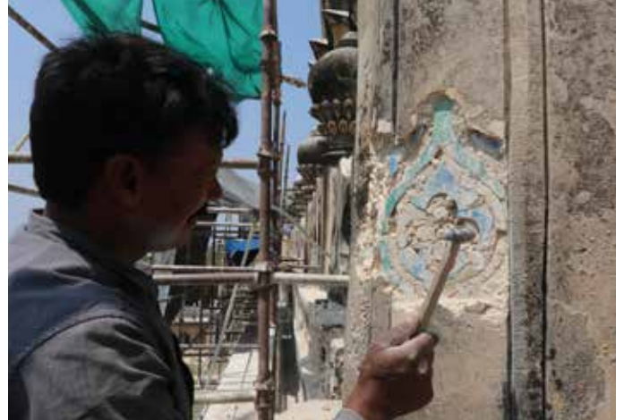
Upon removing the 20 th -century cement plaster, two distinct original multi-colored tiles were discovered on the corner minarets
