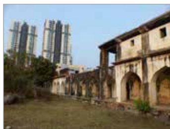
West Elevation - 20th century cement plaster, uneven arch profiles Black Crust, flaking of plaster layer , deteriorated plaster layer, water seepage, missing lime stucco details, missing chajja stone, missing and damaged parapet
