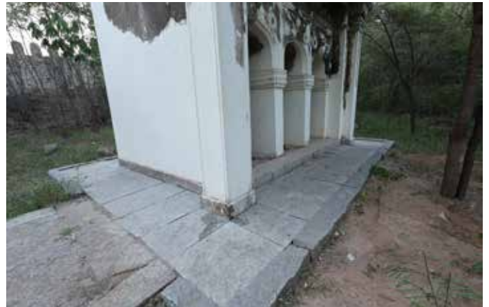
(Left) The grave located close to the monument was repaired and consolidated; (Right) 900 mm wide plinth protection installed around the monument with appropriate slopes to ensure drainage of rainwater away from the monument
