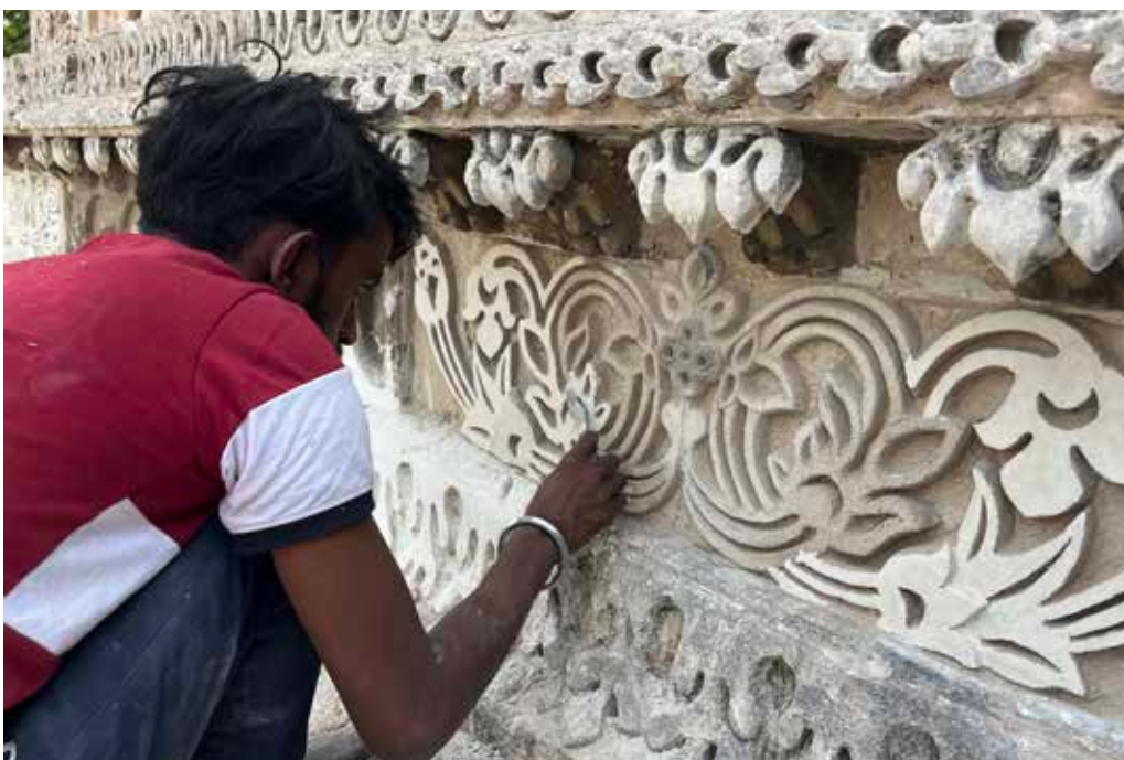
Taking cues from the archival image, master craftspeople skillfully recreated the parapet's original design using traditional materials, replacing the pre-cast cement panels
