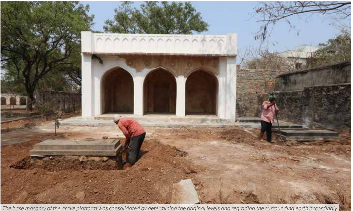
Basework using stone masonry for plinth protection
