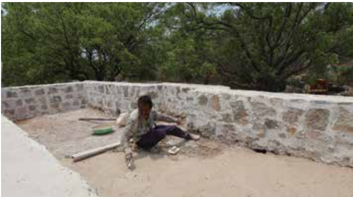
Traditional lime concrete laid on terrace replacing the 20 th century cement
