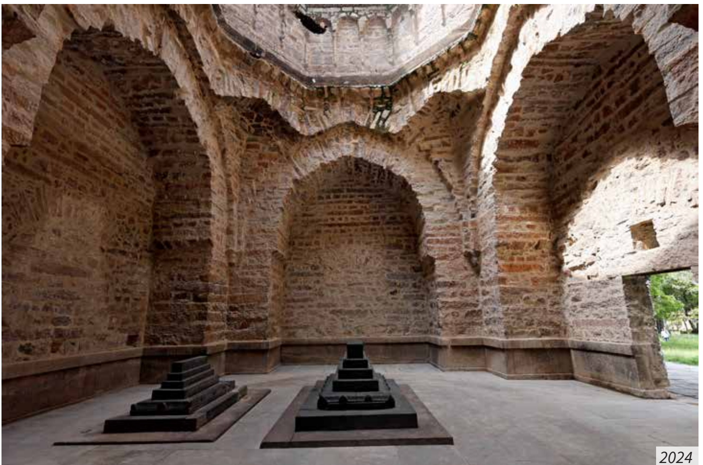
Internal walls of the mausoleum: the 20 th century cement plaster was carefully dismantled to reveal and consolidate the original masonry with lime mortar. The damaged flooring was replaced with a traditional lime concrete base, finished with polished granite stone to ensure durability and proper drainage.
