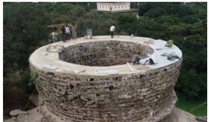
Finishing of the incomplete dome masonry with 20 mm thick granite stone slabs as coping to prevent water ingress and vegetation growth
