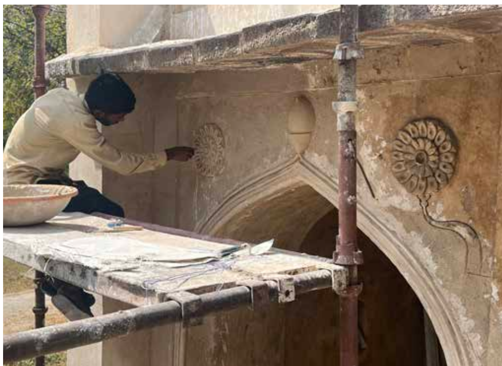
(Top) Removal of inappropriate 20 th century cement plaster from the facade;
