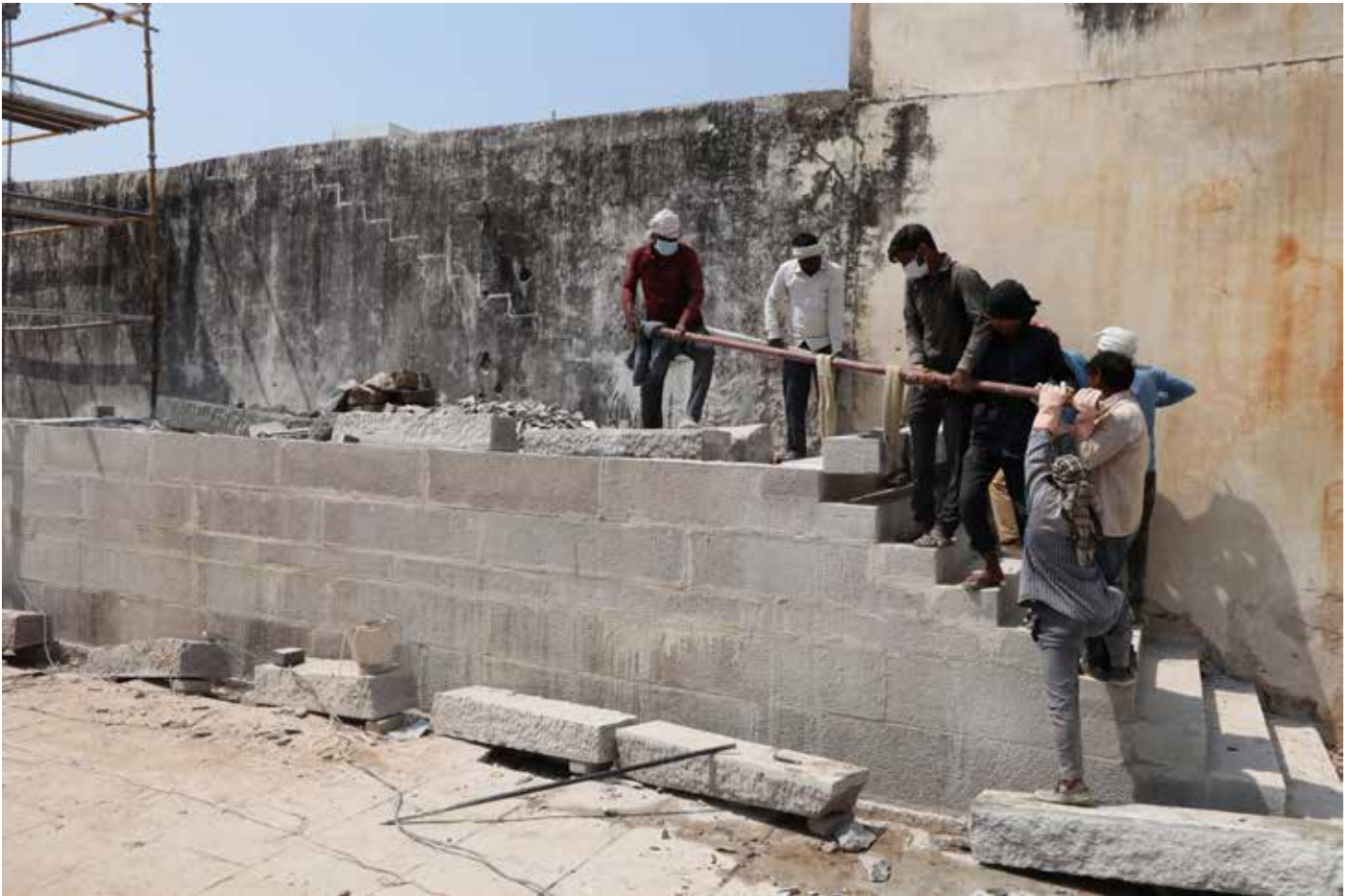
(Clockwise from left) Skilled stone masons prepared hand-chiseled stone blocks for reinstatement at the parapet level and for the staircase; The plinth protection was carefully relaid at original levels in an appropriate slope; Stone craftspeople painstakingly installed a 1.8-meter-wide staircase with 6-inch-thick hand-dressed granite steps to provide access to the terrace/first floor level of the Sarai
