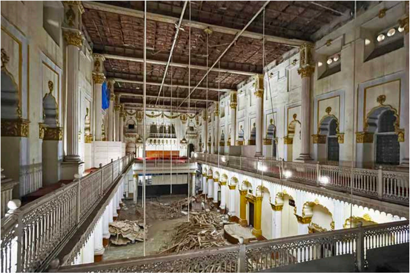
View of the Main Hall after dismantling of later added asbestos ceiling, revealing the historic jack arch ceiling
