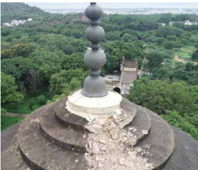
Plaster from the rings on the dome at the finial's base had come loose
