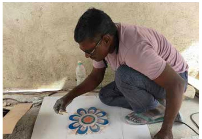
Master craftspeople carefully cut each tile to shape and size, creating samples of the motifs based on the formwork and scaled drawing, ensuring they match the original details revealed
