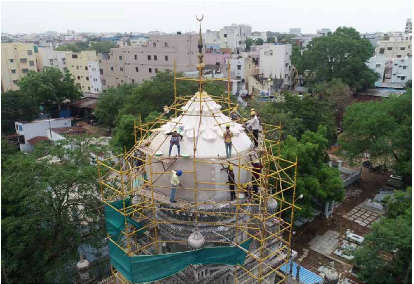
Final lime punning of the dome was completed after surface repairs and replastering
