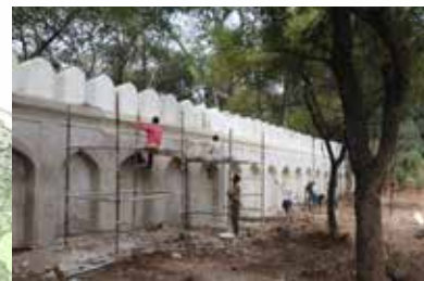
Lime repairs on the arcaded wall
