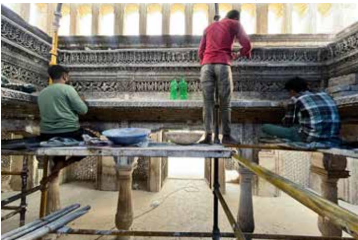
The intricate details at the monuments were minutely cleaned, and the damaged plain and decorative surfaces were carefully restored
