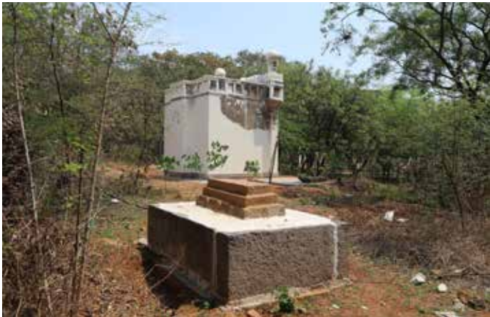
(Left) The grave located close to the monument was repaired and consolidated; (Right) 900 mm wide plinth protection installed around the monument with appropriate slopes to ensure drainage of rainwater away from the monument
