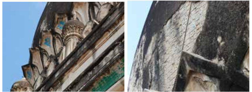
Even before conservation, evidence of 16 th century tiles was visible under the cement covering the mausoleum
