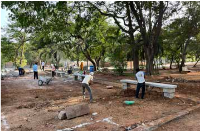
Levelling of earth at a gradual slope for laying of flooring
