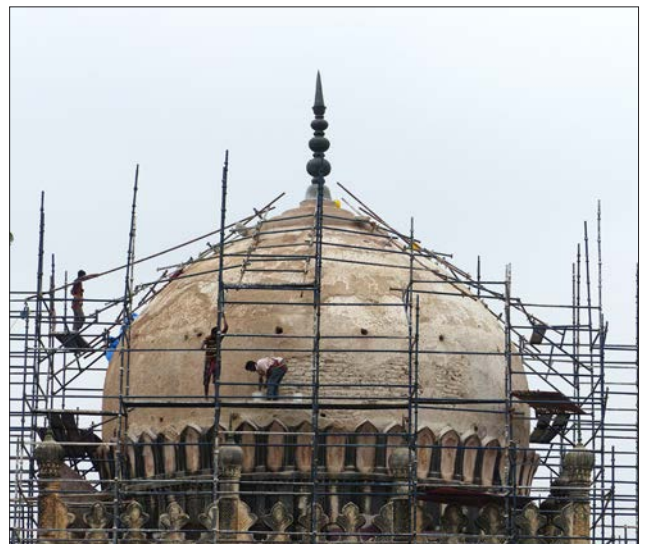
(Left) 6" thick layer of modern plaster with brick infill was removed from the dome prior to replacing with lime plaster
