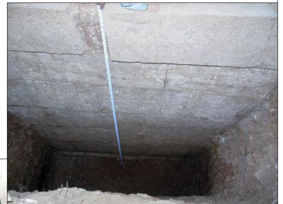
(Left) Excavations unearthed enclosure wall for this tomb on all four sides, giving evidence of the garden enclosure which will be restored. At places, the depth of wall goes down to 7ft from the present ground level.
