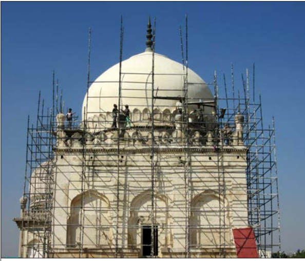
(Left) 20 th century cement plaster from the dome and walls will be removed and replaced with a traditional lime plaster
