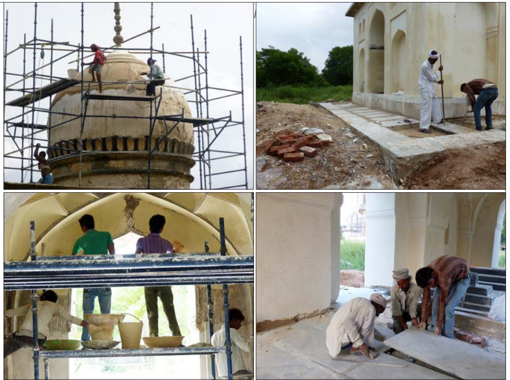
A: Replastering dome in lime mortar; B: Adding granite plinth protection; C: Replastering internal surfaces with lime plaster; D: Cement flooring replaced with stone
