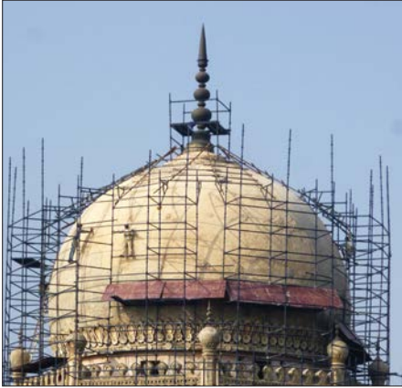
Removal of Cement Plaster
