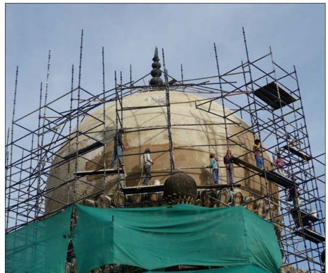
(Left) Removal of cement mortar from the dome (Right) prior to replastering with lime mortar
