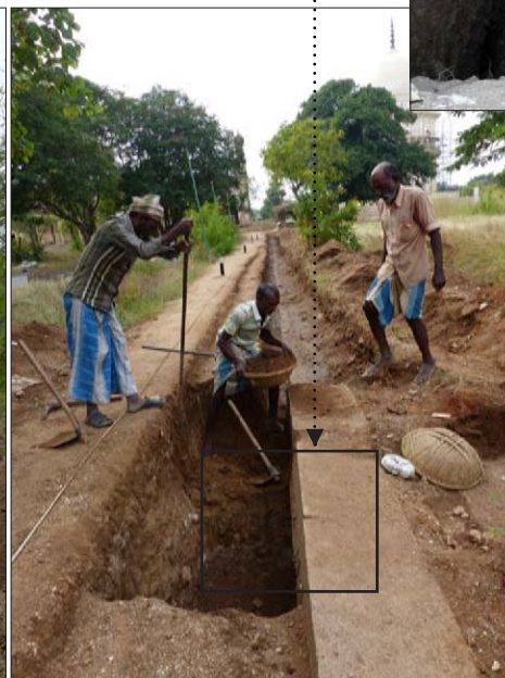
(Left) Excavations unearthed enclosure wall for this tomb on all four sides, giving evidence of the garden enclosure which will be restored. At places, the depth of wall goes down to 7ft from the present ground level.
