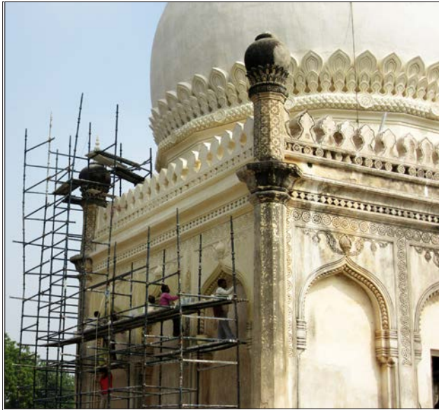
(Above) Replastering and repairing of the exteriors
