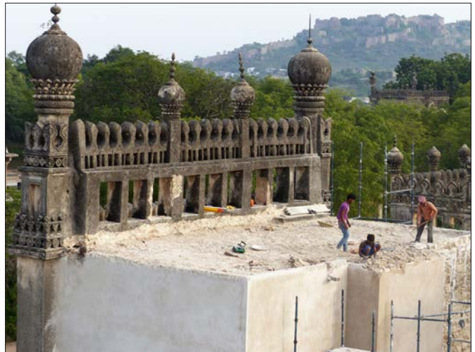
(Above) The external surface plaster was dismantled and fresh lime plaster was applied to the rear, north and south sides
