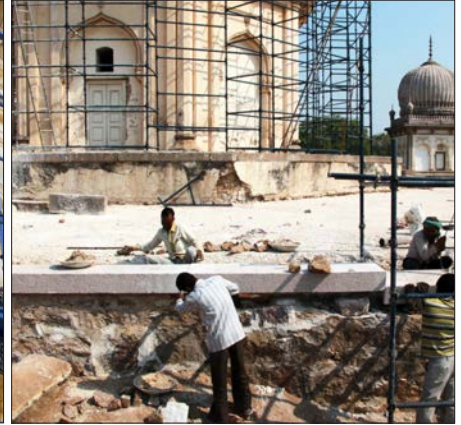
Installing Stone Edging on Plinth
