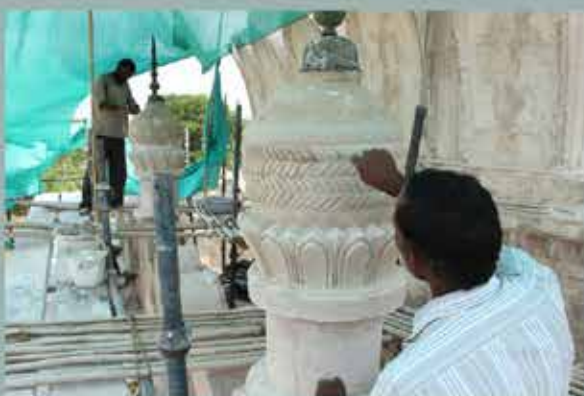
Discovery of these patterns in-situ allowed a scientific restoration of the patterns where these were missing. Restoring historic details using traditional techniques and materials.
