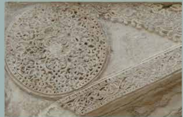
This revealed intricate stucco medallions and arch crowns on the North facade. Similar patterns were found on the arched openings.
