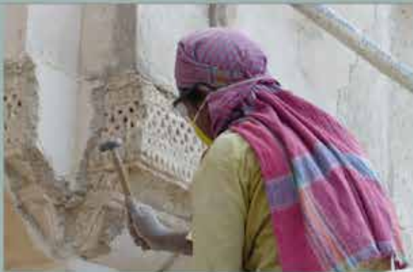
As part of the conservation efforts, several layers of cement, which were added during 20 th century repairs, were removed.
