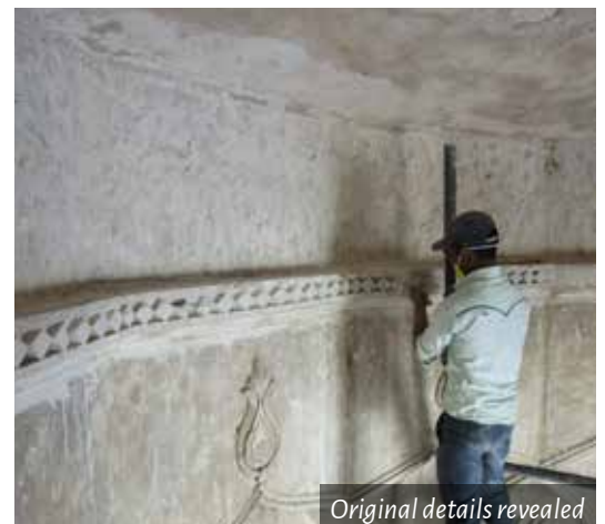
Final layer of lime mortar being applied on the facade
