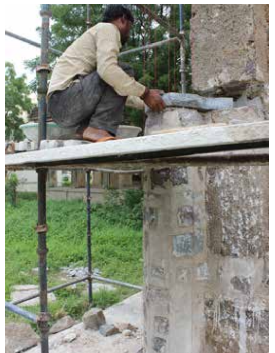
(Middle ) Restored facade of the mausoleum; (Bottom) Reconstruction of the octagonal profile corner pier
