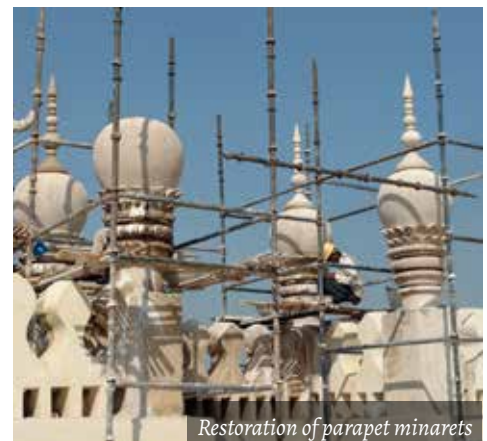
Repairs using lime plaster after removal of cement
