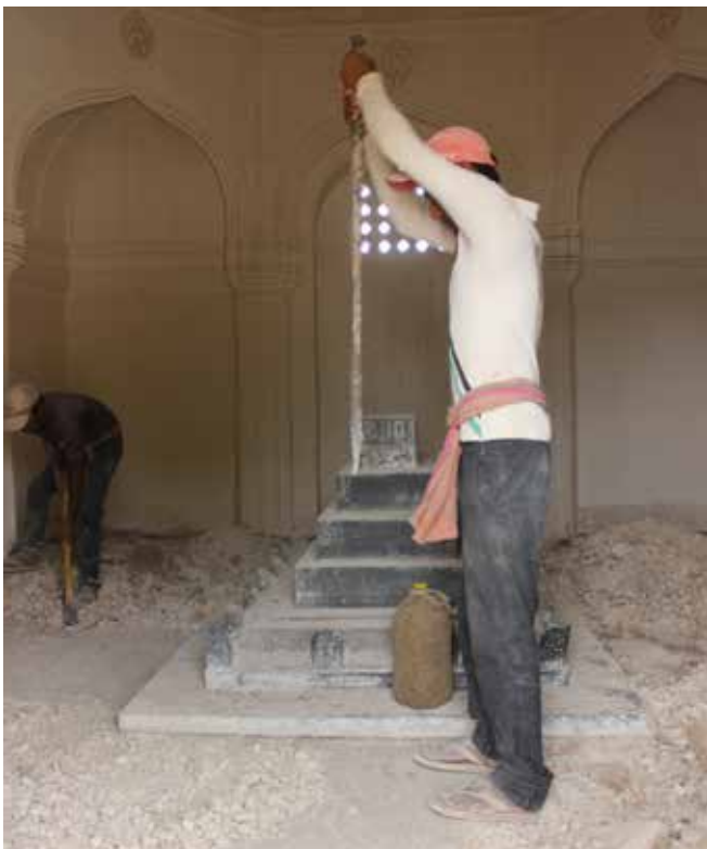
(Left) 20 th century cement flooring was dismantled (Below) Final lime finish of the internal surface
