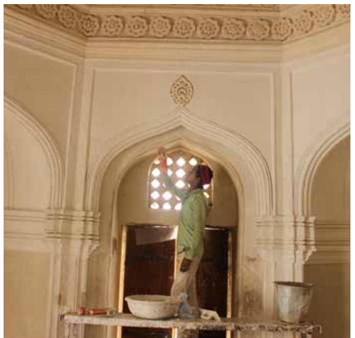
(Left) 20 th century cement flooring was dismantled (Below) Final lime finish of the internal surface
