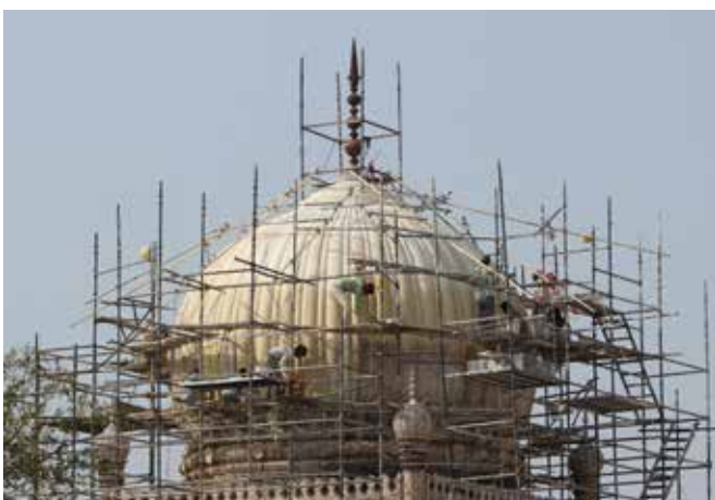
Later added plaster layers from the dome were removed to reveal the original curved profile of the ribs, and repaired using lime mortar
