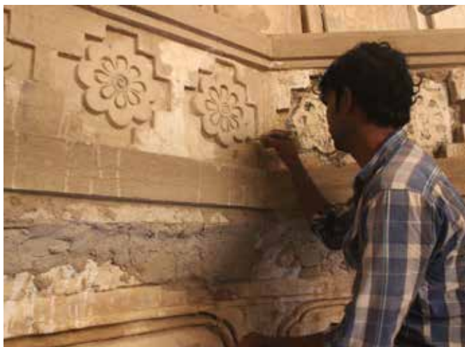
(Left) Restoration of incised lime plaster details on the internal surface; (Right) Final finish with lime punning at the internal portion of the mausoleum
