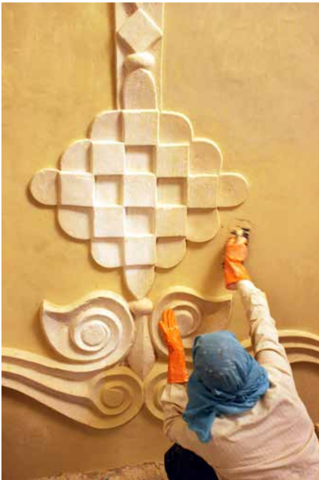
(Left) Final lime punning of the ornamental detail on the internal surface below the dome; (Top Right) The internal dome surface and the ornamental details were carefully cleaned of modern layers and repaired and finished with lime; (Bottom Right) Outline of the original detail found on dismantling of modern plaster layers on internal surfaces
