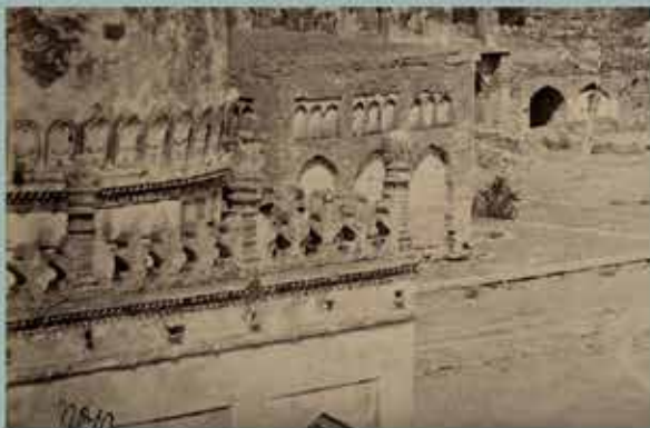
The archival images of 1860s depicted the tomb's external surface to be covered with ornate lime stucco works on the walls. The arches were crowned with medallions. The minarets had ribbed plaster and the merlons were studded with highly ornate lime stucco.
