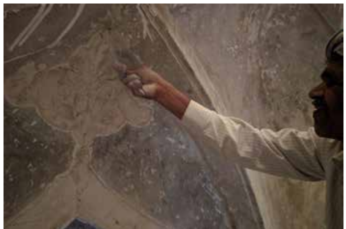
(Left) Final lime punning of the ornamental detail on the internal surface below the dome; (Top Right) The internal dome surface and the ornamental details were carefully cleaned of modern layers and repaired and finished with lime; (Bottom Right) Outline of the original detail found on dismantling of modern plaster layers on internal surfaces
