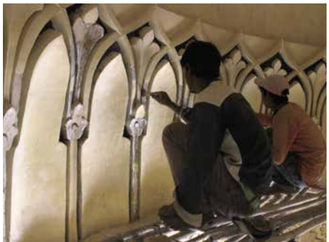
(Left) Restoration of incised lime plaster details on the internal surface; (Right) Final finish with lime punning at the internal portion of the mausoleum
