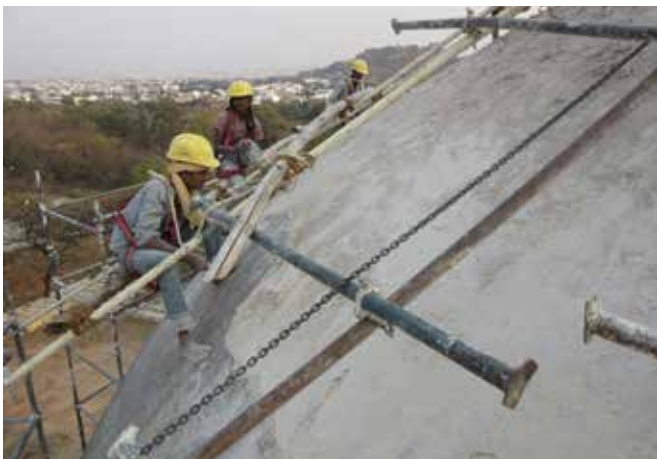
Dismantling of damaged and loose cement plaster from the dome 20 th century cement and brick paving abutting the main cenotaph removed
