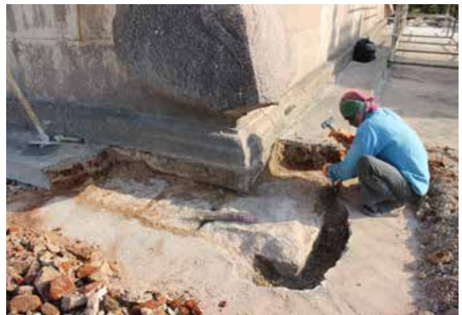
Dismantling of damaged and loose cement plaster from the dome 20 th century cement and brick paving abutting the main cenotaph removed
