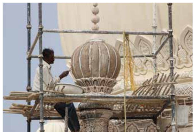
The cemented portions of minars were removed and repaired in lime mortar
