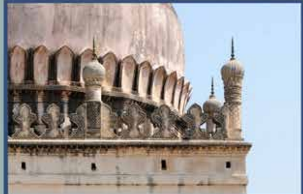
However, mid-20 th century repairs had obfuscated original details and the tomb was found covered with a layer of cement plaster
