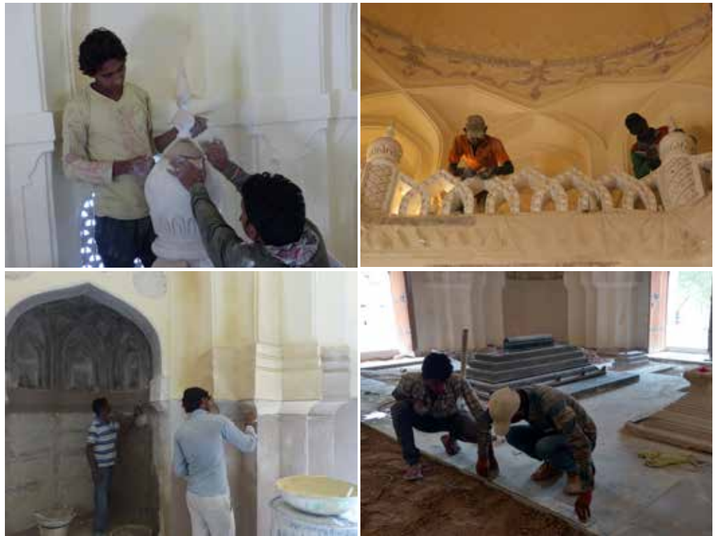
(Clockwise from left) Missing finials on minarets reconstructed using lime mortar; later added lime wash was scrapped off from the intersecting arches above the gallery level to reveal the original profile and ornamentation; rich lime mortar applied on the entire internal surface after necessary repairs to the existing details; 30 mm thick granite stone slabs laid to appropriate slope and approved pattern
