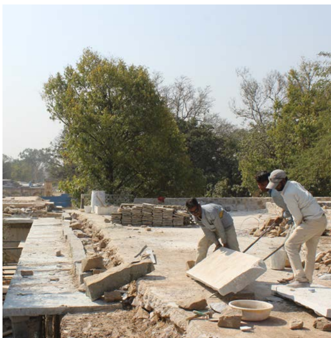
Stone eaves installed on the facade of serai
