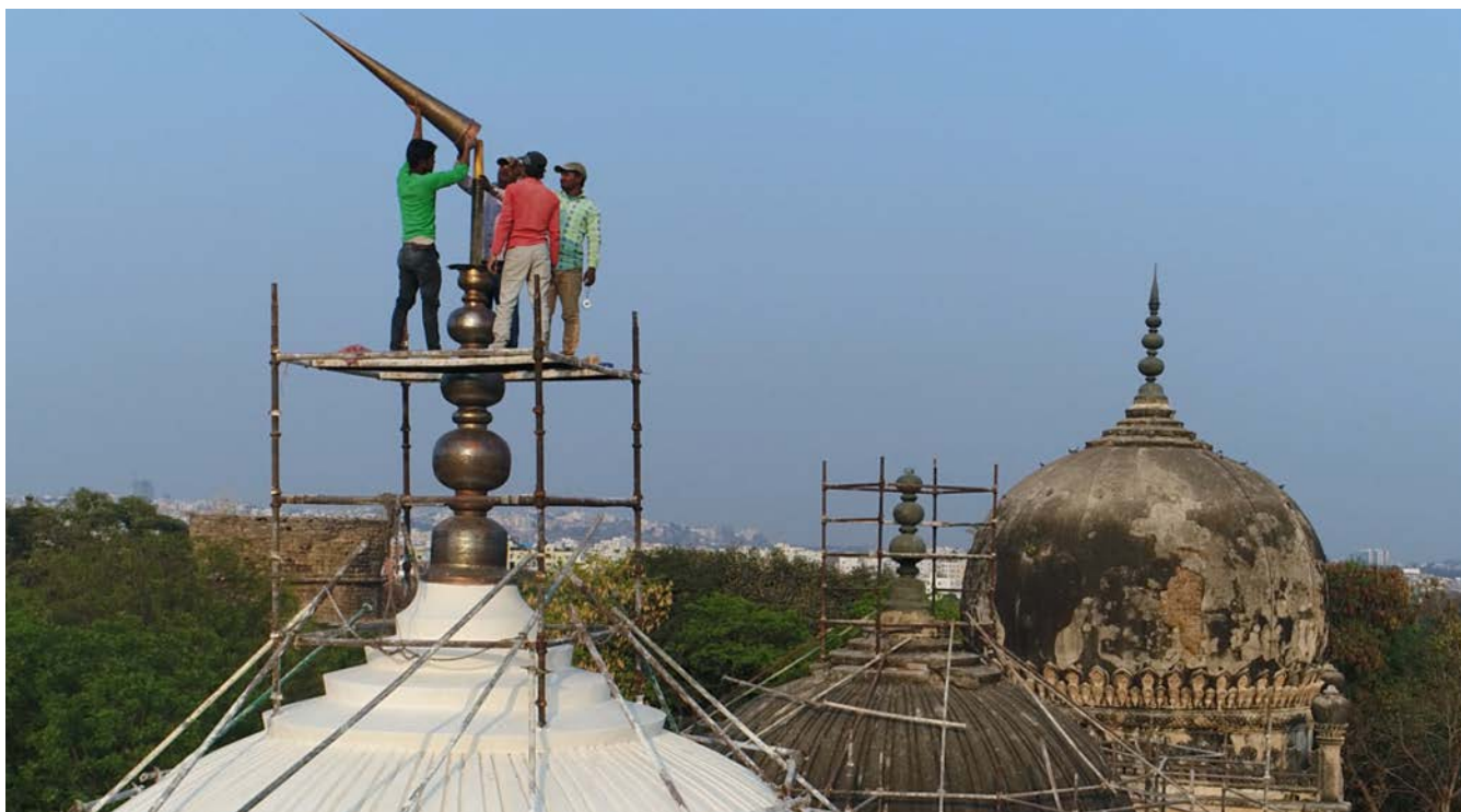
Installation of finial on the western dome of the twin mausoleums of Hakims'. (Top Left) Cement finial on the mausoleum to the west ; (Top Right) Local coppersmith fabricating components of copper finial; (Below) Installation of the finial on the dome
