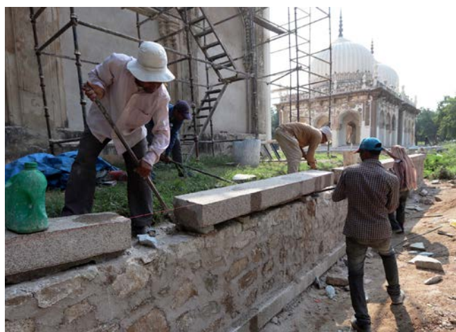
The plinth wall at Commander's mausoleum was bulging due to water ingress, was hence dismantled and followed by reconstruction with stone and lime mortar and installation of hand-chiseled stone coping
