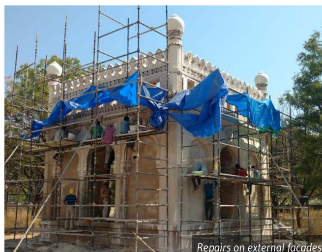
Restoration of ornamental details in arch crowns
