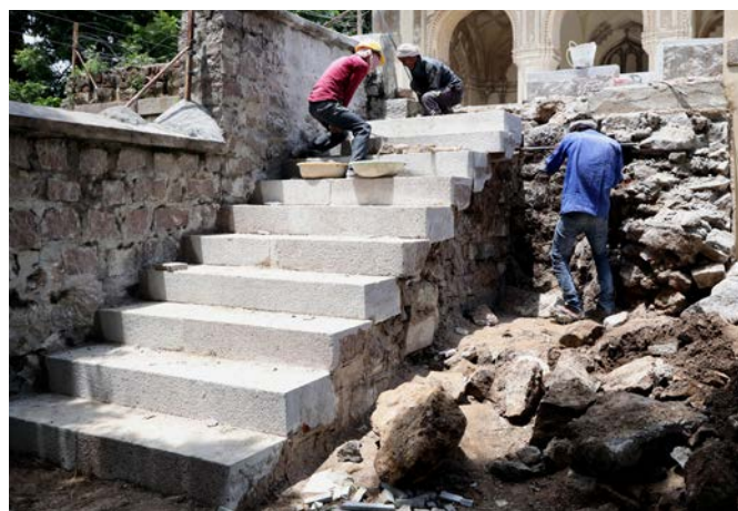
(Left) Restoration of lime stucco details on the facade; (Top Right) Installation of granite stone edging around the 'wazu'tank; (Bottom Right) Installation of hand chiseled dressed stone steps
