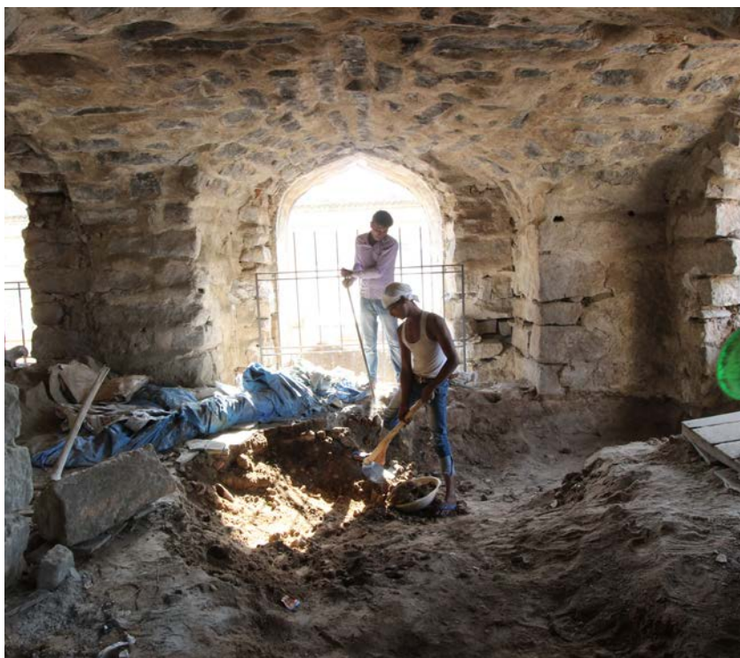
(Left) Removal of excess earth and debris; (Top Right) Lime concreting for installation of flooring; (Bottom Right) 30 mm thick granite stones laid
