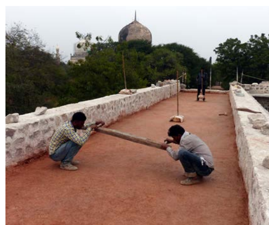
(Left) Reconstruction of arcade using traditional honeycomb shuttering (Top right) Installation of stone beams on the reconstructed arcade's roof; (Bottom right) Ramming of the lime concrete laid on top of the stone beams
