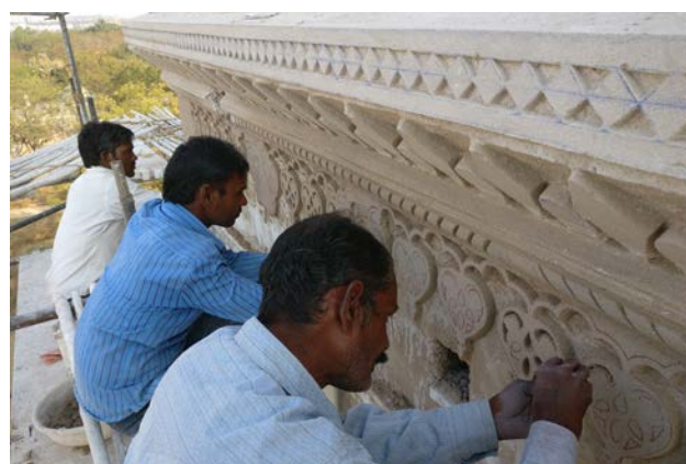
Conservation works were preceded by removing cement layers to reveal hidden tiles and stucco work - all of which have been well documented and consolidated to prevent ingress of water
