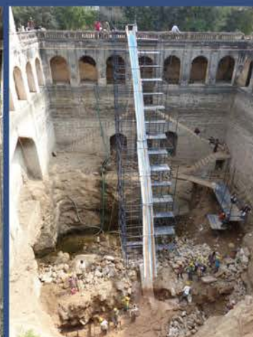
Construction of retaining wall using traditional lime mortar
