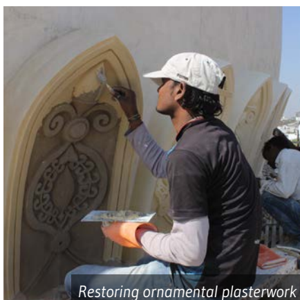
Removal of damaged and loose plaster layers
