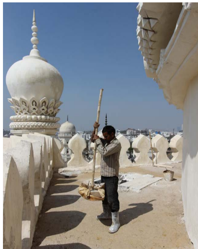
The cement from the roof was replaced with traditional lime mortar
