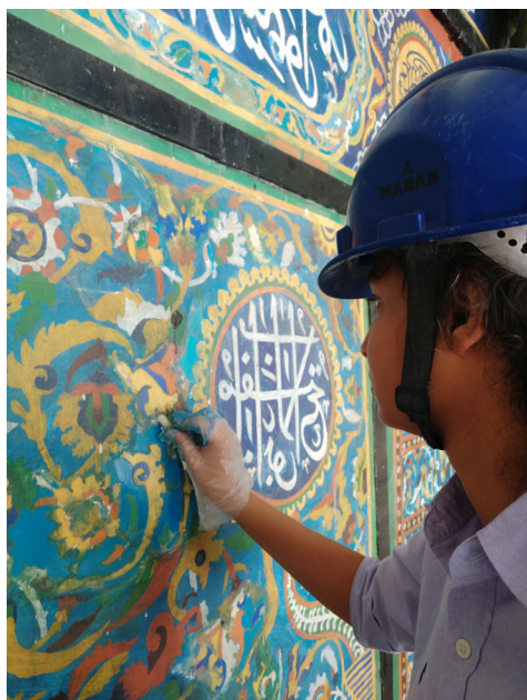
Removing paint layers to reveal the original enamelled tile underneath.
