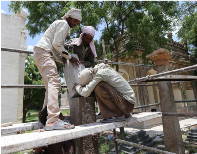
A hand carved stone piece of matching profile was retrofitted with stainless steel dowels along with epoxy resin
