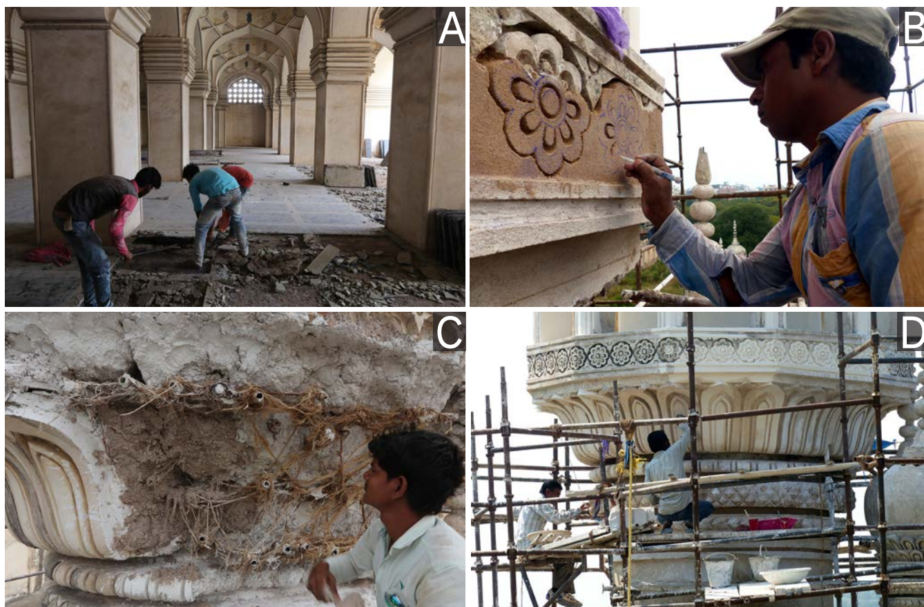
A: Dismantling of inappropriate 20 th century stone flooring; B: Carving of floral medallions by lime craftsman ; C: Reinforcing damaged portion of minarets with jute fiber and lime mortar; D: Finishing of restored floral brackets supporting the arch gallery
