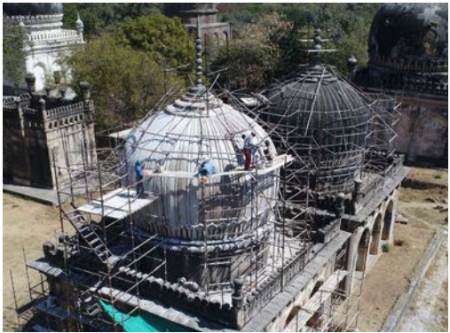
(Above) Restoration of the ribs on the dome of Hakims mausoleum in lime mortar
