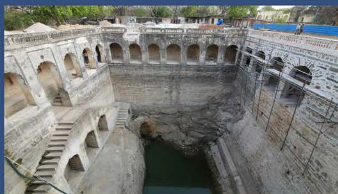
Existing stones from the collapsed western wall reused for repair of the wall.
