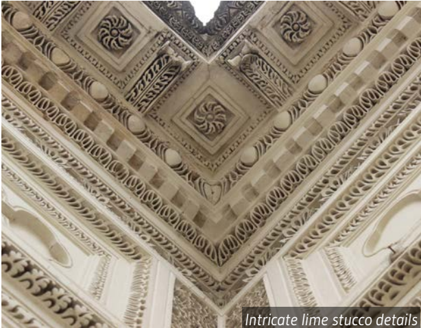
Intricate lime stucco details
