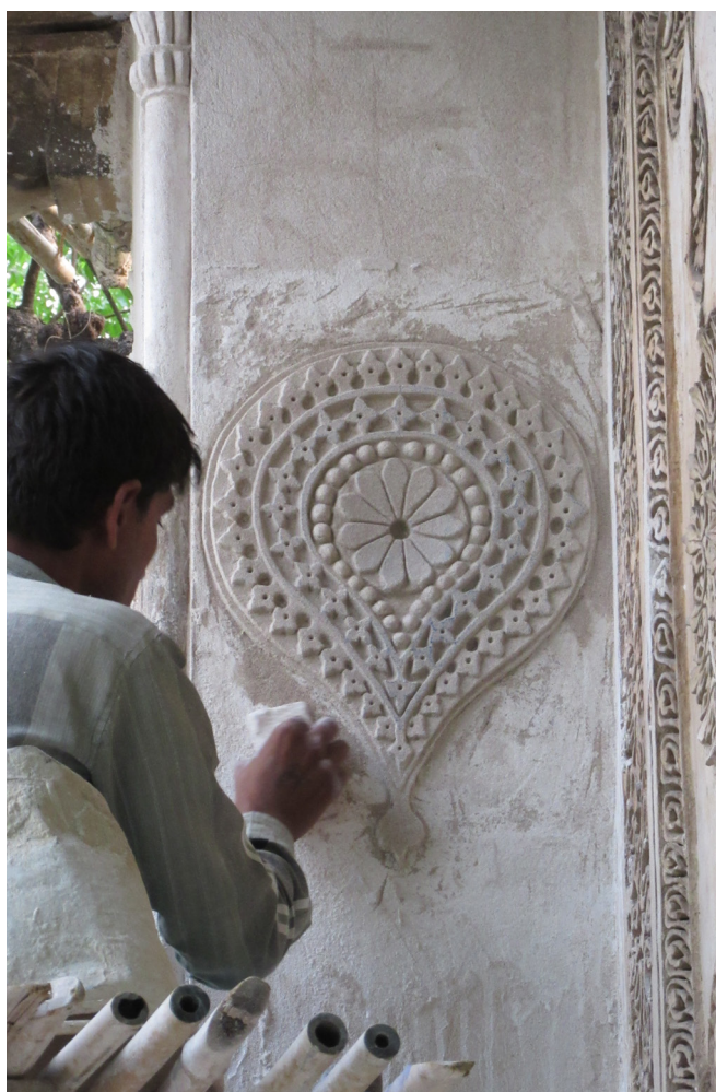
(Left) Restoration of lime stucco details on the facade; (Top Right) Installation of granite stone edging around the 'wazu'tank; (Bottom Right) Installation of hand chiseled dressed stone steps
