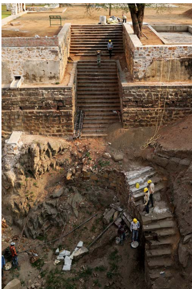
Repairs of the steps carried out, missing steps were reinstated
