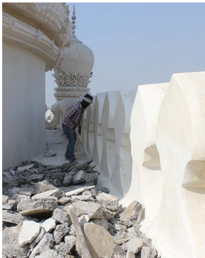
Removal of 20 th century cement layers from the roof of the mausoleum
