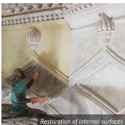
Removal of damaged and loose plaster layers
