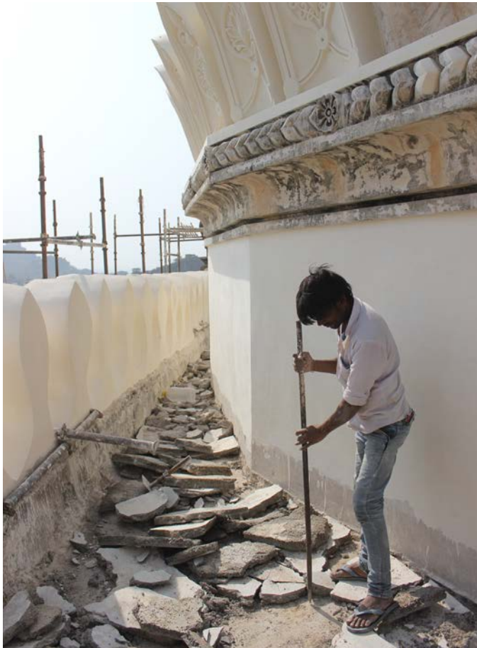
Removal of 20 th century cement concrete layers from the terrace of the mausoleum
