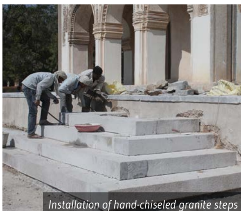
Installation of 30 mm thick granite stone slabs
