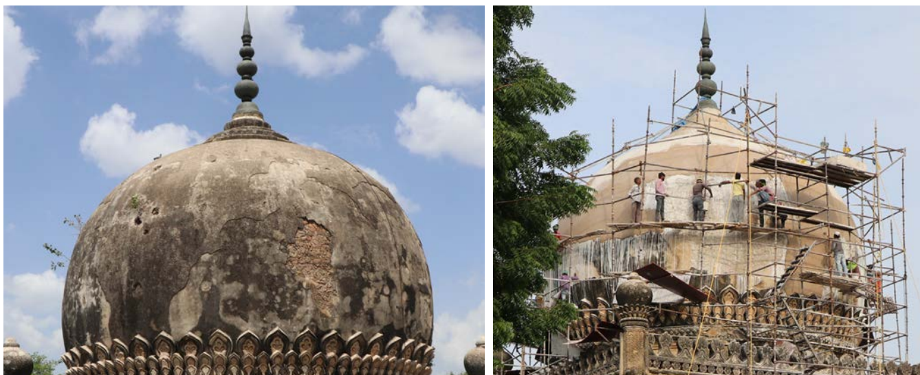
(Left) The dome of the mausoleum of Commander was covered with 20 th century cement plaster which was causing damage; (Right) After careful removal of the cement layers, lime plaster was applied on the dome.
