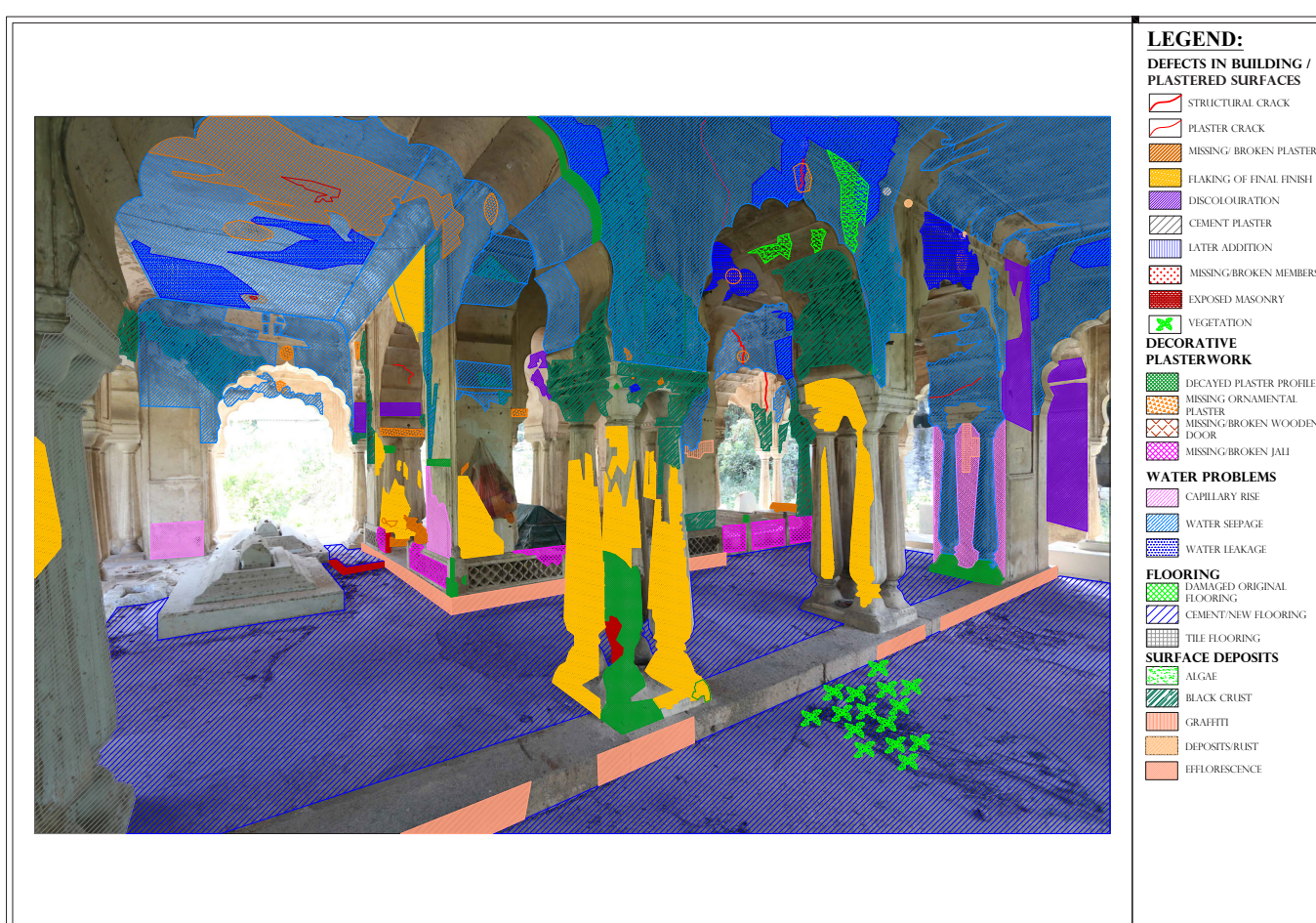
Condition assessment of Mausoleum of Ghansimiyan
