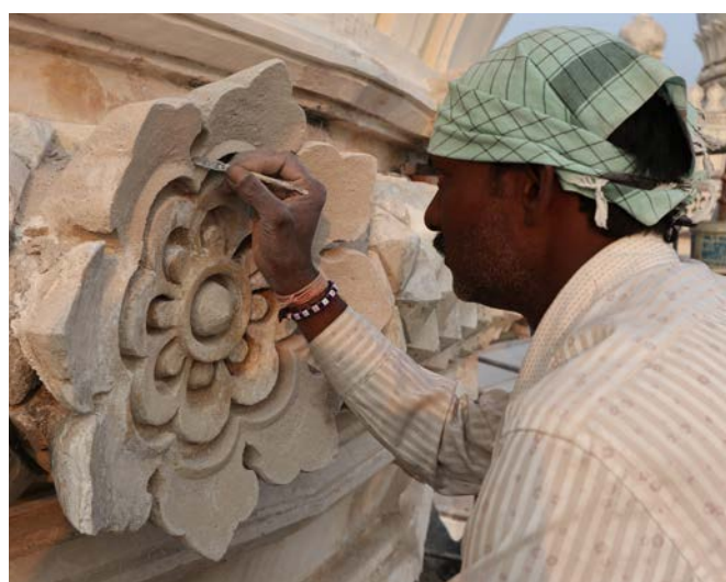
Restoration of ornamental detail
