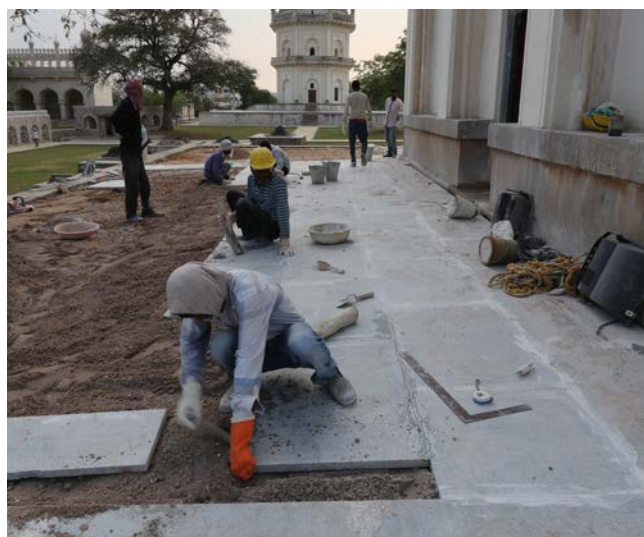
Removal of cement concrete from the plinth to halt further deterioration Laying of stone slabs on a layer of lime mortar to replace the cement
