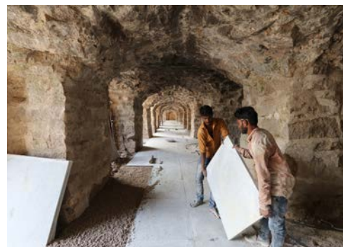
(Left) Removal of excess earth and debris; (Top Right) Lime concreting for installation of flooring; (Bottom Right) 30 mm thick granite stones laid
