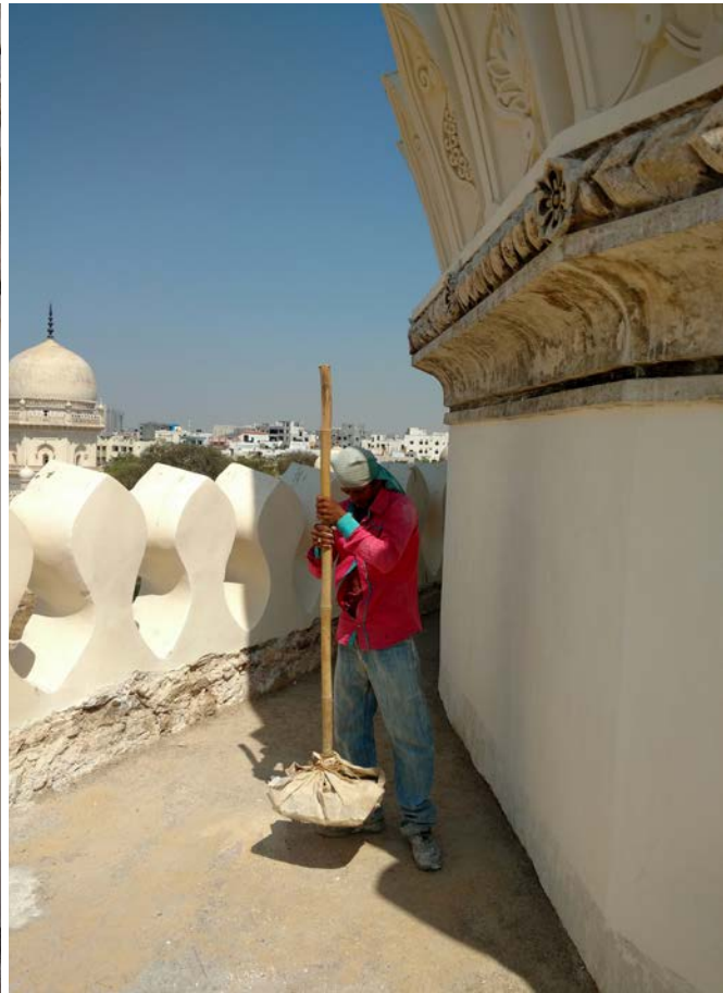
The cement from the terrace was replaced with traditional lime concrete
