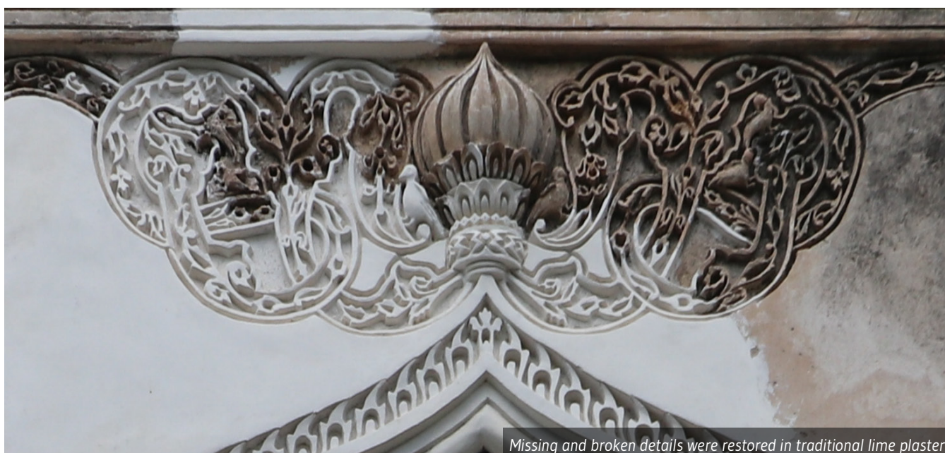
Lime craftsman restoring the ornate stucco detail
