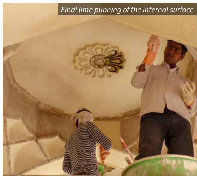
Floral details restored with traditional lime plaster
