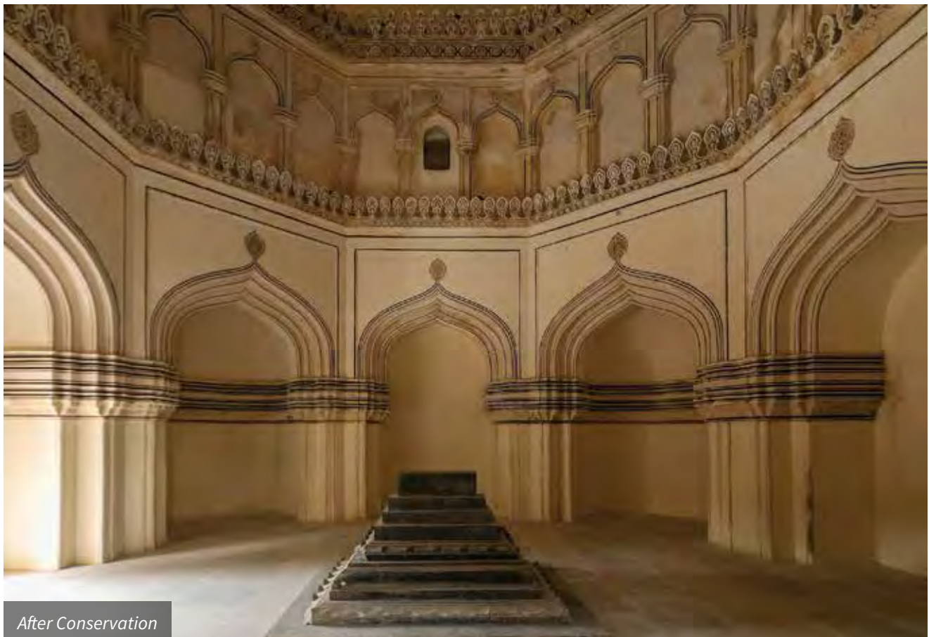
Restoration of capital band in lime plaster
