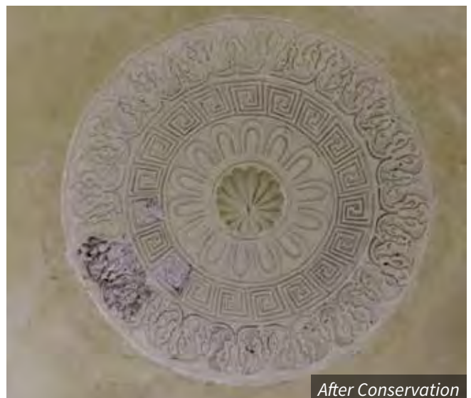
Restoring the ceiling medallion based on in-situ evidence
