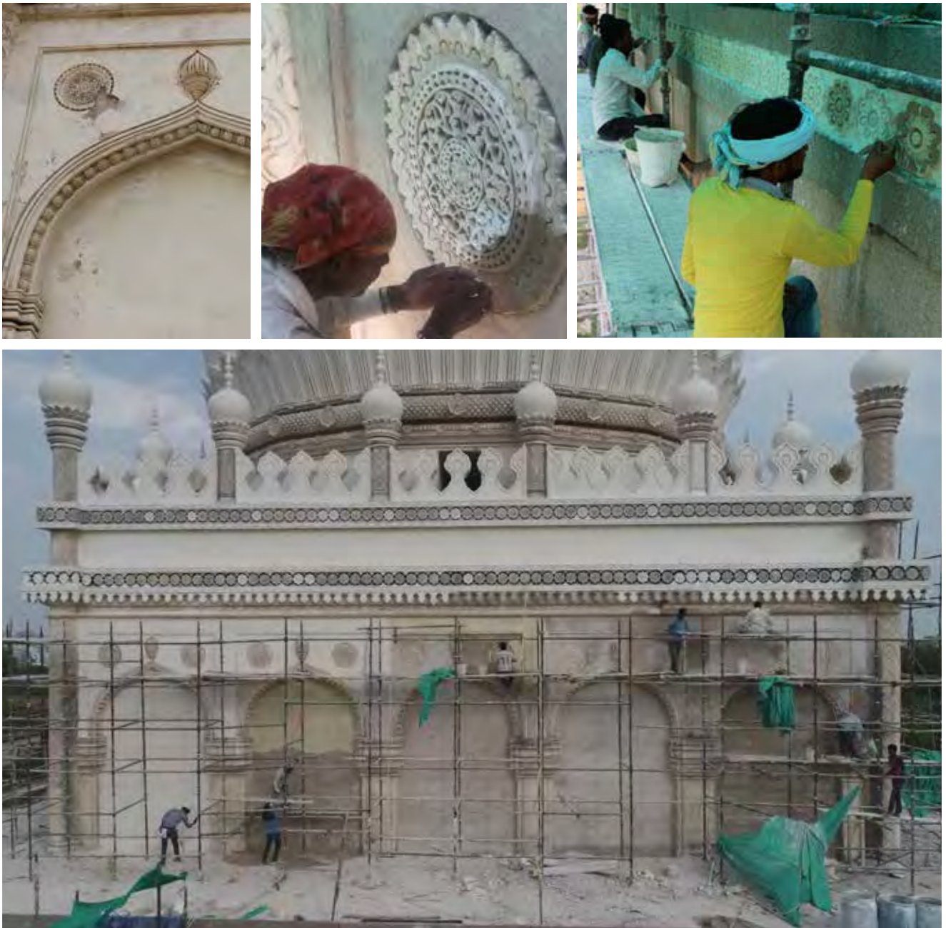
(Above) On the external facade, the broken and damaged ornamental details and architectural elements were repaired and restored using traditional lime plaster and finished with a coat of lime punning based on existing evidence.
