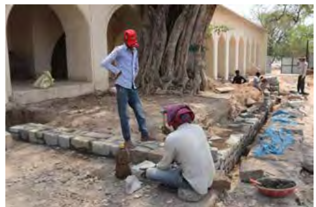
Retaining walls were built around the holding earth of the Peepal tree abutting the monument
