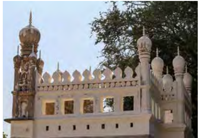
(Clockwise from left) The external facade of the mosque was repaired with lime mortar after removal of 20th century cement and white wash layers; Restoration of decorative plasterwork on parapet; Craftsmen repairing and restoring the battlements
