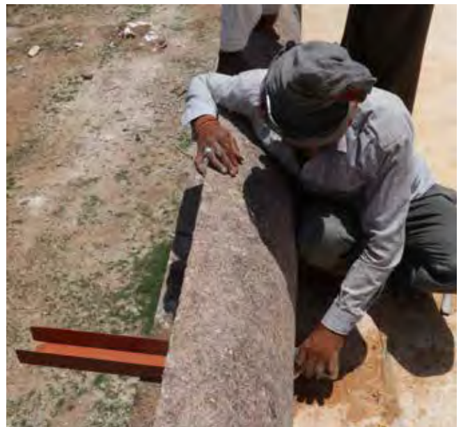
(Above) Stone parapet realigned on the middle terrace, and (Below) Metal water spouts installed in existing openings for a proper drainage of the rainwater.
