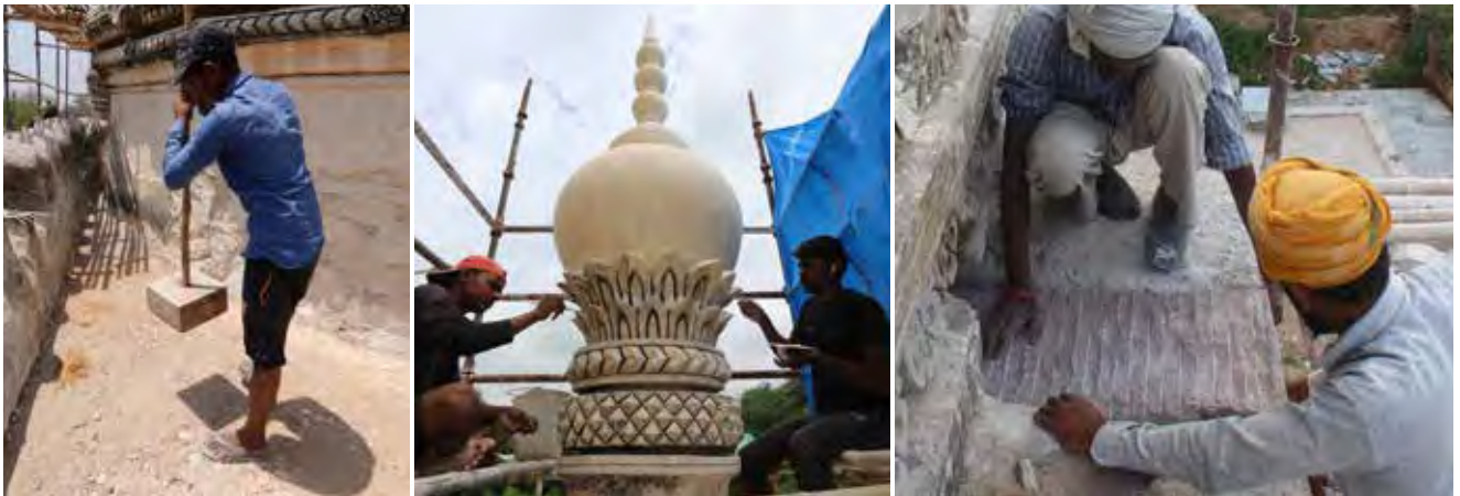
Left - Cement from the terrace was removed and replaced with traditional lime concrete in an appropriate slope
