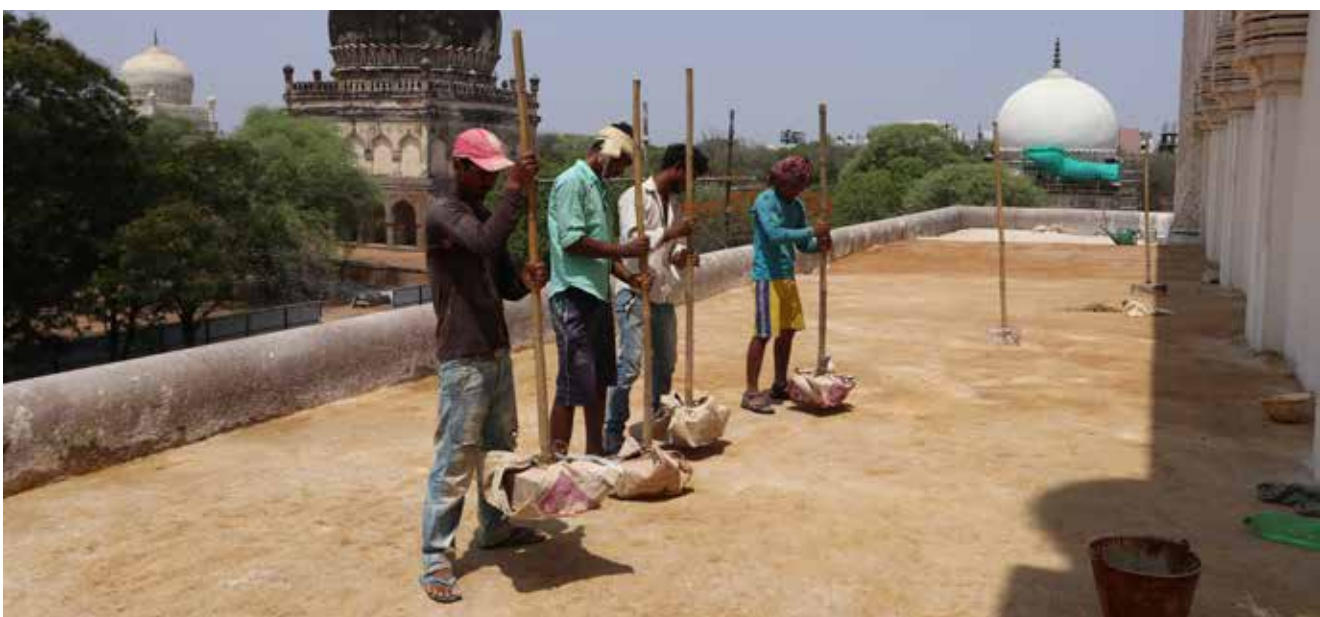
(Above) Dismantling of 20th century cement concrete on the middle terrace; (Below) Traditional lime concrete was laid in appropriate slope
