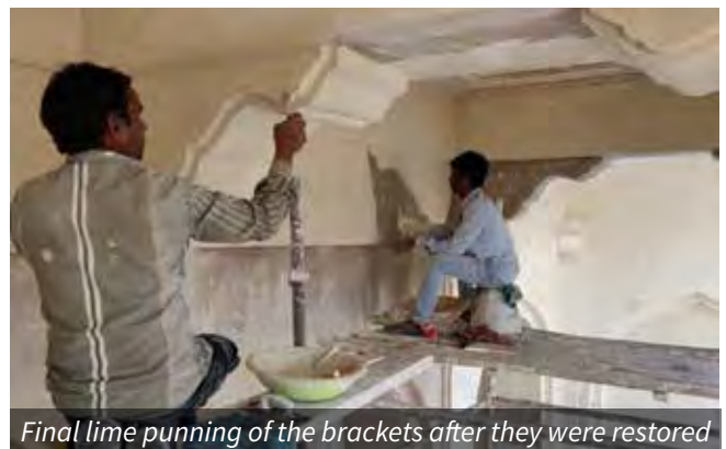
Repairs with traditional lime mortar
