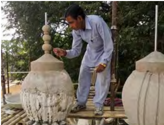
(Top) Restoration of details and minarets on the parapet; (Bottom Left) Repairs on the collapsed portions of a minaret and installation of missing finial on top; (Bottom Right) Missing minarets were restored using traditional lime mortar
