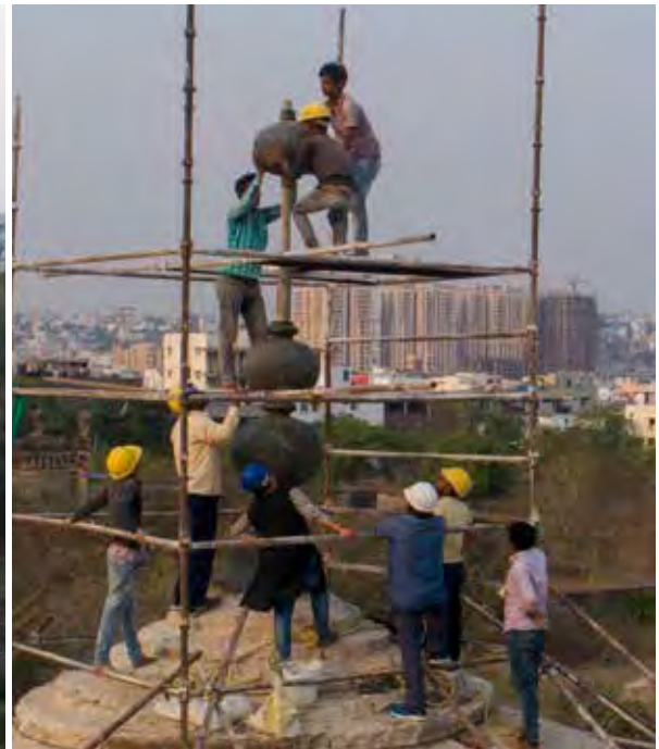
(Left) Before final installation, pieces of the copper finial were assembled on the ground to ensure that the GI pipe inserted in the center fits appropriately; (Right) Installation of the repaired pieces of copper finial atop the dome
