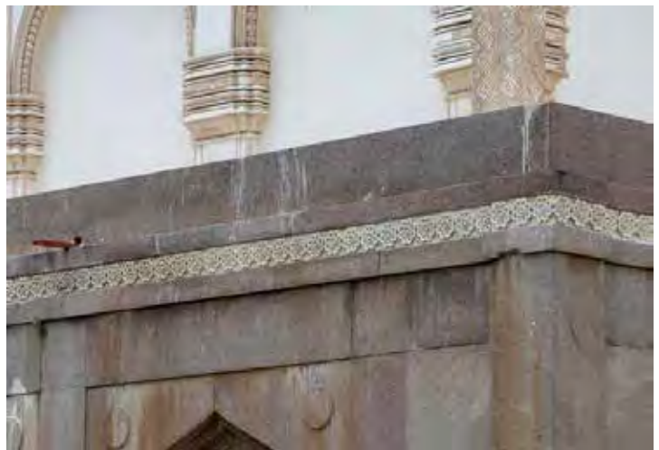
(Above) Stone parapet realigned on the middle terrace, and (Below) Metal water spouts installed in existing openings for a proper drainage of the rainwater.
