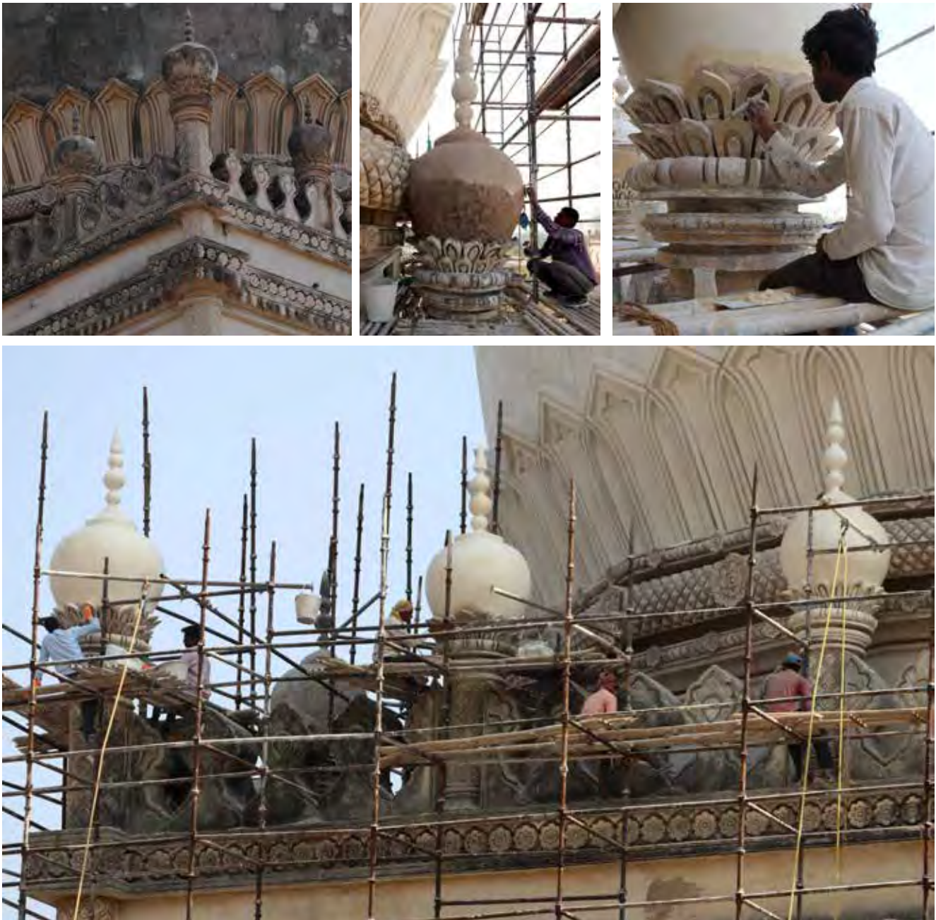
(Above) Cement layers from the minars were removed and replaced with traditional lime plaster, missing and broken details were restored and damaged finials were re-installed.
