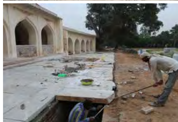
6.4 meters wide plinth protection was finished with 100 mm thick natural rough granite stones with the grading towards the aqueduct. Care was taken that the historic water channel running at the south of Hamam is not affected and is being covered with granite stone slabs
