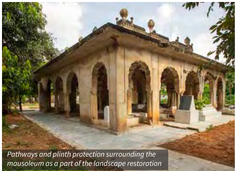
Re-installation of broken minarets on the parapet of the mausoleum
