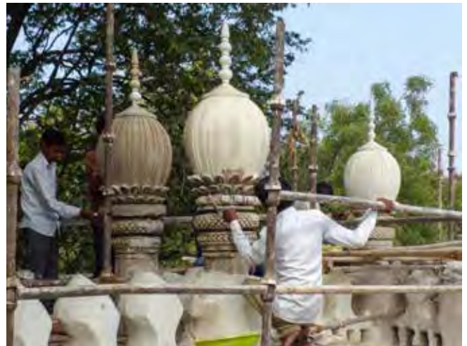
(Top) Restoration of details and minarets on the parapet; (Bottom Left) Repairs on the collapsed portions of a minaret and installation of missing finial on top; (Bottom Right) Missing minarets were restored using traditional lime mortar
