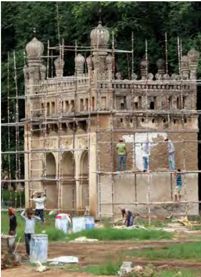
(Clockwise from left) The external facade of the mosque was repaired with lime mortar after removal of 20th century cement and white wash layers; Restoration of decorative plasterwork on parapet; Craftsmen repairing and restoring the battlements
