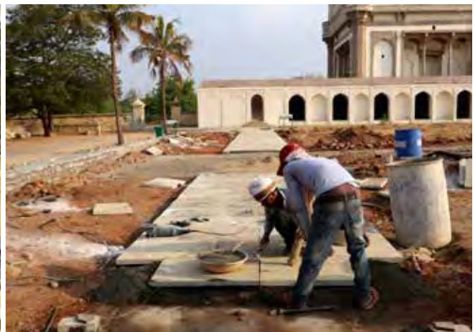
(Left) Construction of plinth wall along the raised forecourt; (Right) Installation of paving stone on the pathways constructed as a part of the landscape master plan
