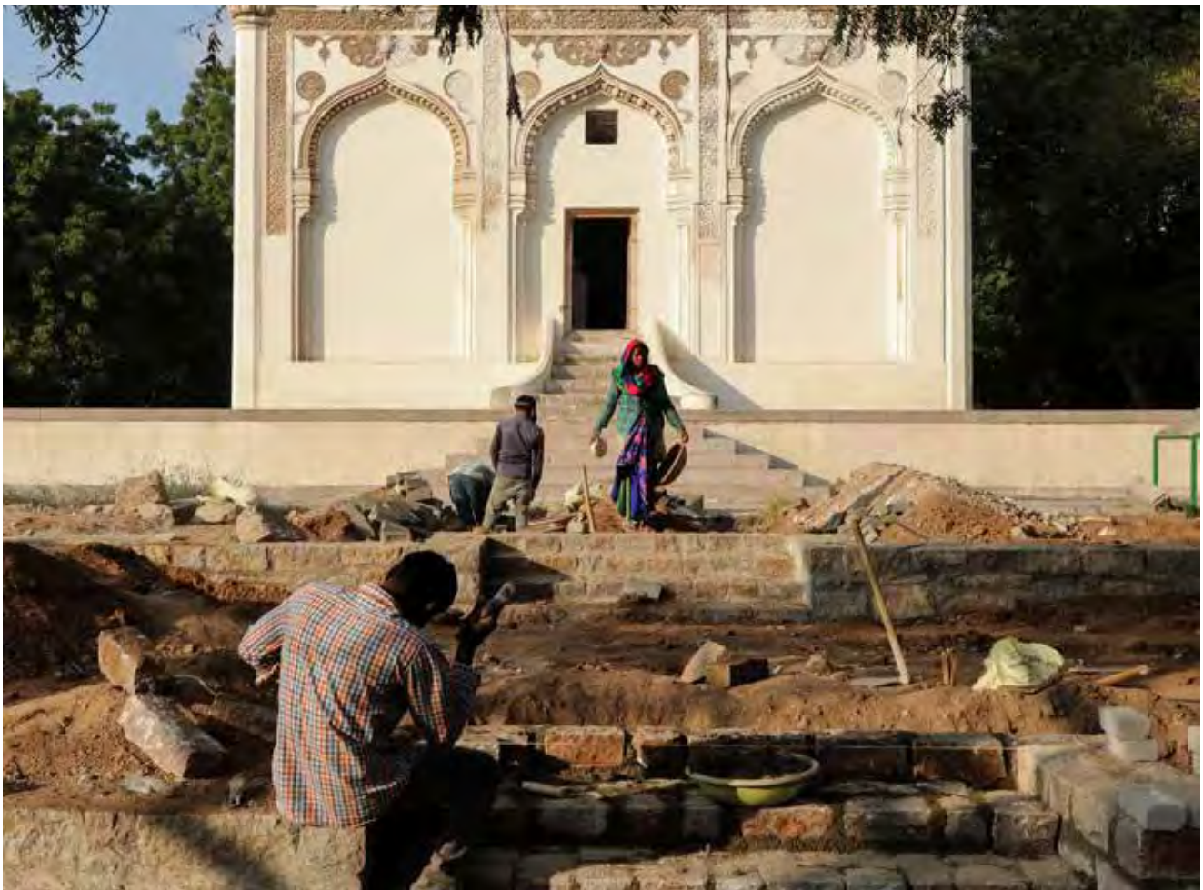
(Top) Pathways were built connecting Fatima's mausoleum to Commander's mausoleum; (Bottom) Construction of steps as part of the plaza south of Commander's mausoleum
