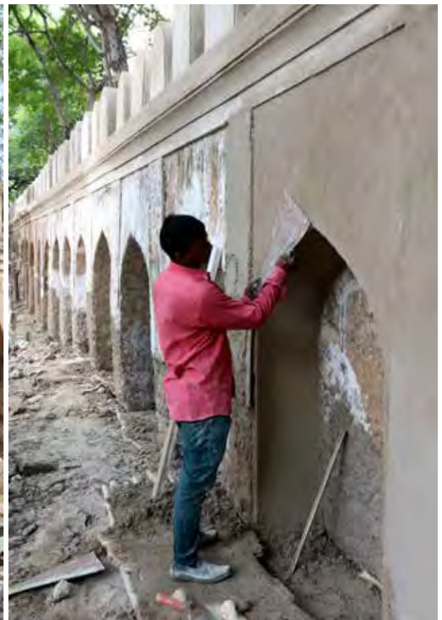
Replastering of the wall surface and repairs on the arches using traditional lime mortar
