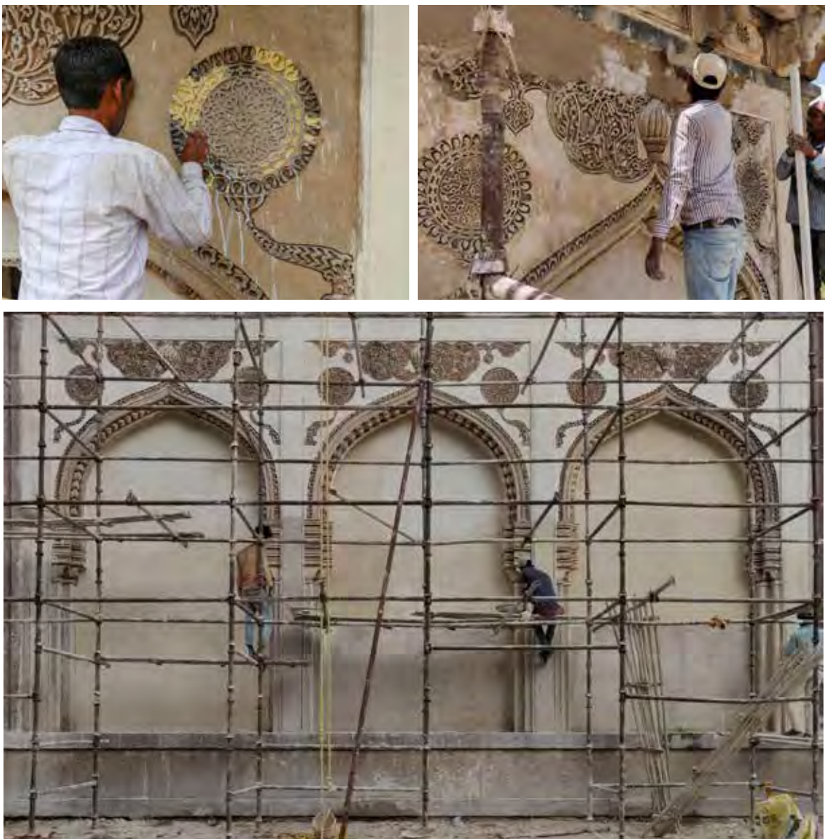
Missing and damaged ornate stucco patterns on the external facade of the mausoleum were carefully restored by craftsmen
