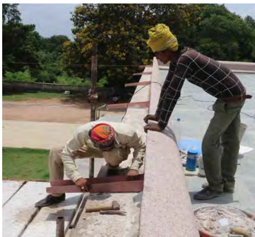
(Clockwise from left) Installation of metal waterspout on the parapet at upper plinth; Grouting and pointing with lime mortar on all the joints at the upper plinth level; Cleaning of existing rainwater spouts
