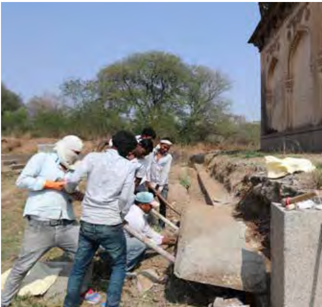
Stone craftsmen fixing the hand chiselled granite blocks lining the plinth of Premamati's mausoleum.
