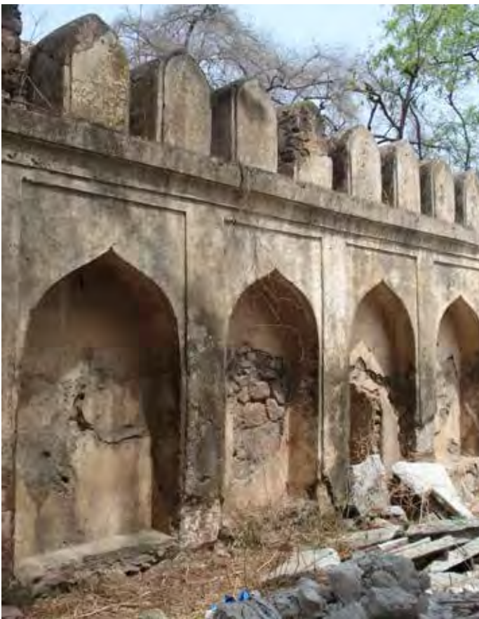
Removal of 20th century cement and damaged plaster from the wall surface
