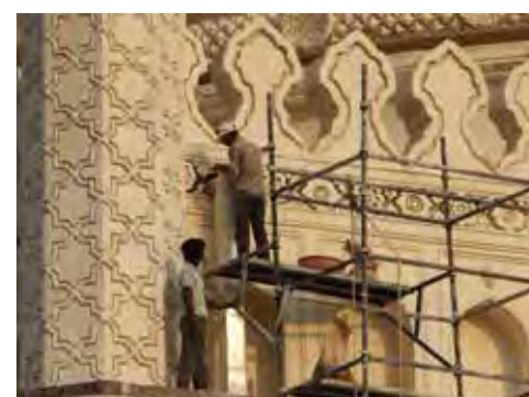
(Clockwise from left) Installation of metal waterspout on the parapet at upper plinth; Grouting and pointing with lime mortar on all the joints at the upper plinth level; Cleaning of existing rainwater spouts
