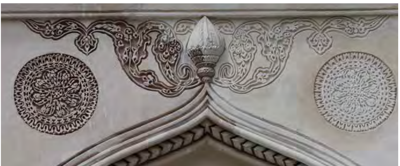
20 th century cement repairs on the decorative elements on the spandrel were carefully dismantled, and restored in traditional lime mortar as per site evidence
