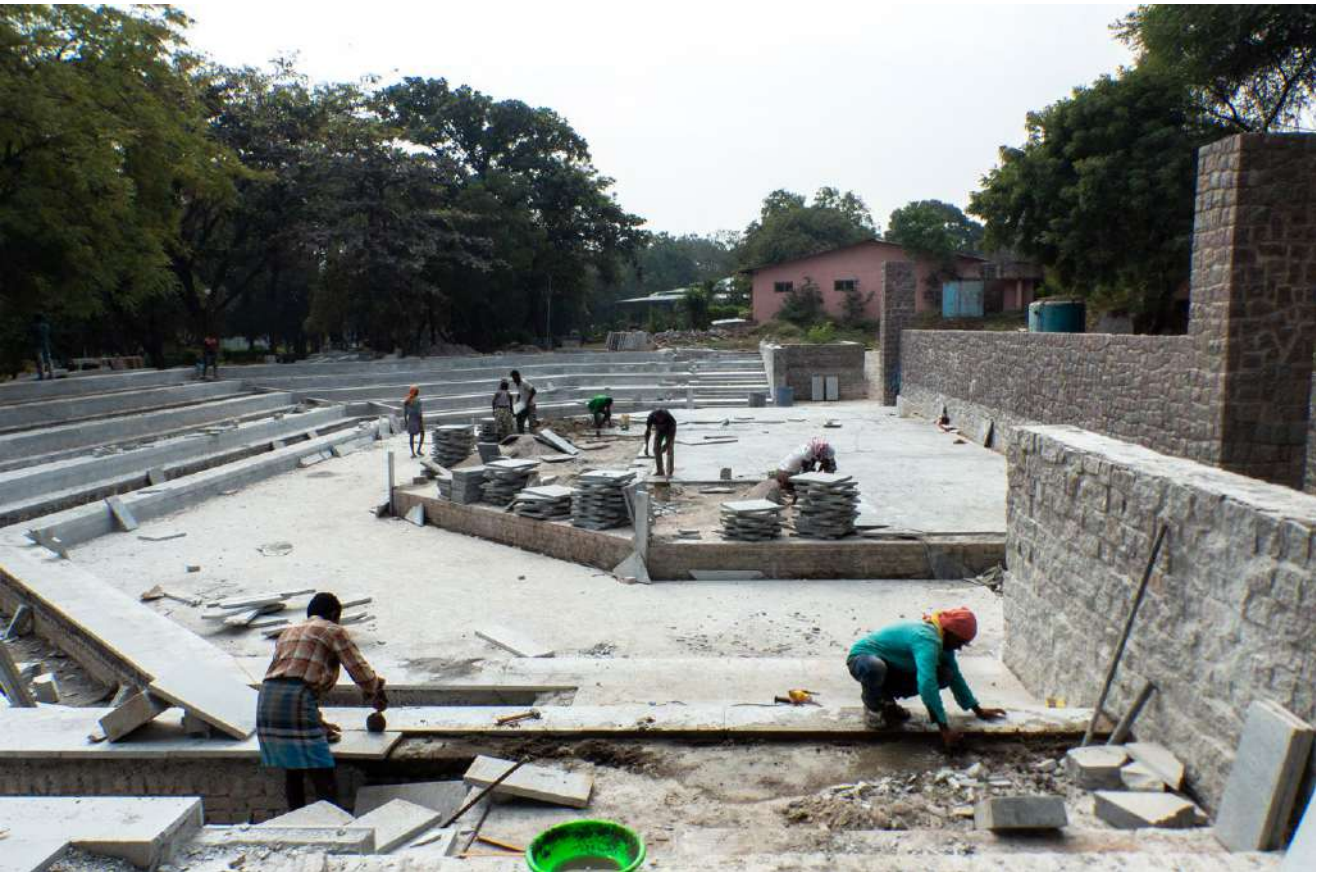
(Left) Tying of Reinforcement mats for the car parking area before laying of final road finish; (Below) Construction of stone steps and the stage area at the amphitheater
