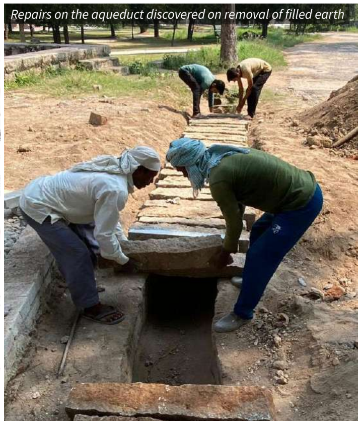
6.4 meters wide plinth protection was finished with 100 mm thick natural rough granite stones with the grading towards the aqueduct. Care was taken that the historic water channel running at the south of Hamam is not affected and is being covered with granite stone slabs
