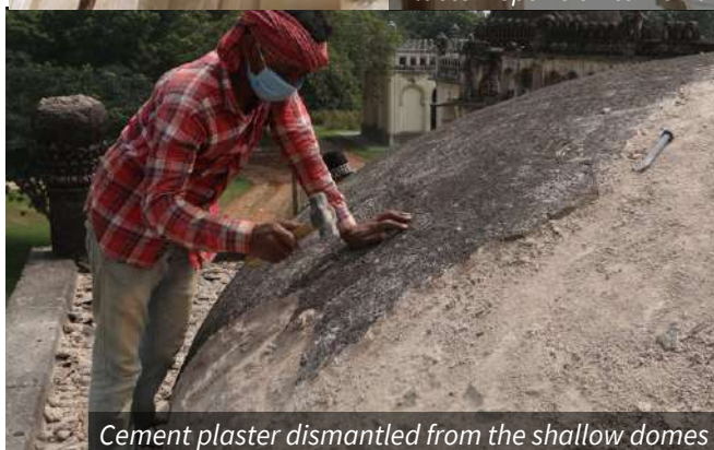
Plaster repairs on tomb 10
