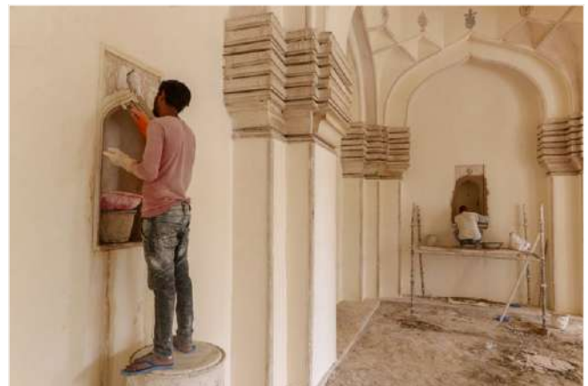
Ornamental stucco details were restored on the internal wall surfaces
