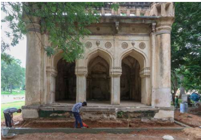
Stone craftsmen installed a plinth protection around the funerary mosque
