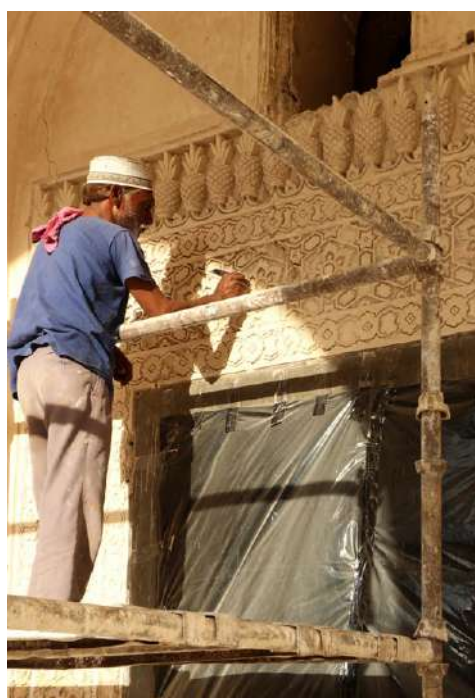
(Right) Ornamental stucco frieze around the stone doorway jambs were meticulously restored by skilled craftsmen based on original evidence
