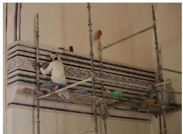
Ornamental stucco details and moulding bands were restored inside the internal mausoleum matching the existing evidence
