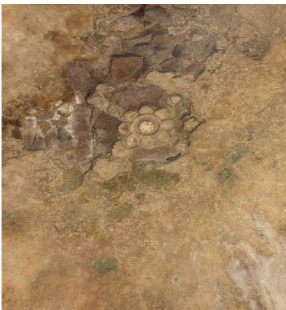
Mastercraftsmen reinstating ornamental stucco ceiling medallion at a tomb using rich lime mortar. A true size stencil was made based on the existing evidence, and the design was transferred onto lime plaster for restoration of damaged portions
