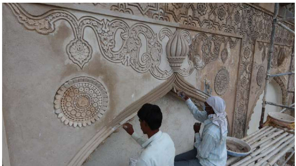
(Above) Restoration of original ornamental stucco medallions underneath the projected eaves below the terrace carried out by traditional lime craftsmen; (Below) Moulding bands, ornamental stucco and arch crowns restored using traditional lime mortar
