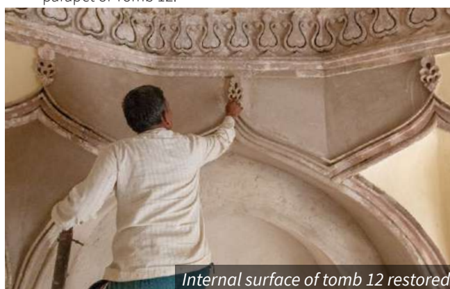
Plaster repairs on tomb 10
