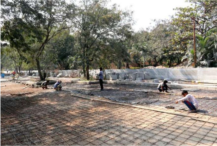
(Left) Tying of Reinforcement mats for the car parking area before laying of final road finish; (Below) Construction of stone steps and the stage area at the amphitheater
