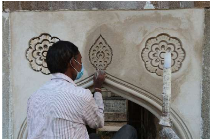
(Left) Plaster repairs were carried out at the internal surface of the tomb; (Right) Missing details on the facade were restored based on in-situ evidence
