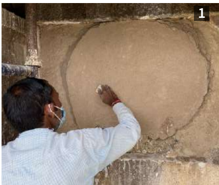
(Above) Restoration of original ornamental stucco medallions underneath the projected eaves below the terrace carried out by traditional lime craftsmen; (Below) Moulding bands, ornamental stucco and arch crowns restored using traditional lime mortar
