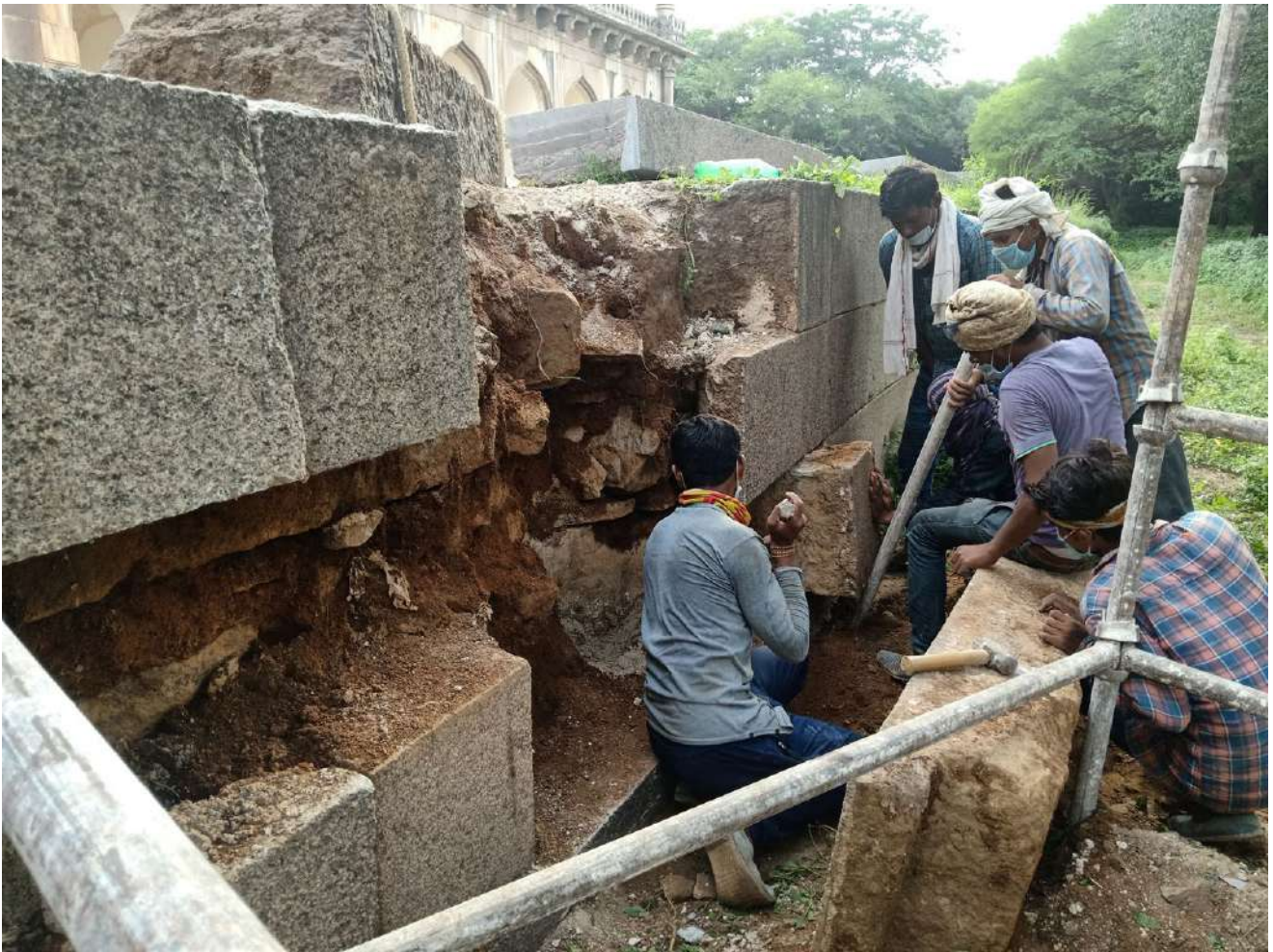
Realignment of the stones lining the plinth wall as per original design
