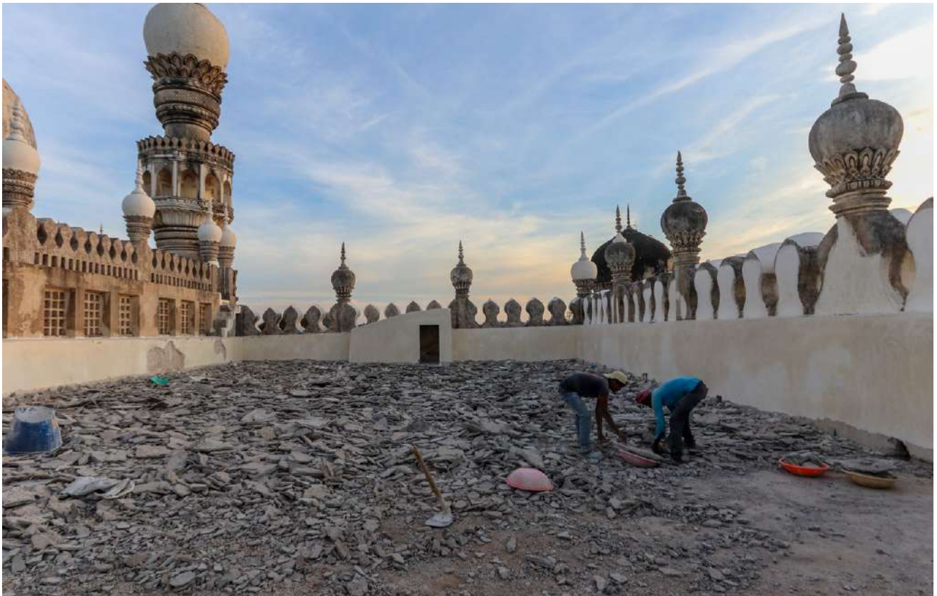
(Above) Dismantling of 20th century cement concrete on the middle terrace; (Below) Traditional lime concrete was laid in appropriate slope
