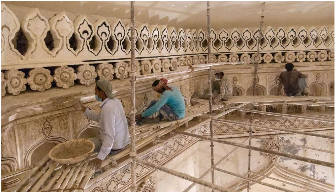
(Above) Ornamental moulding bands situated above the projected arch gallery were restored using lime mortar
