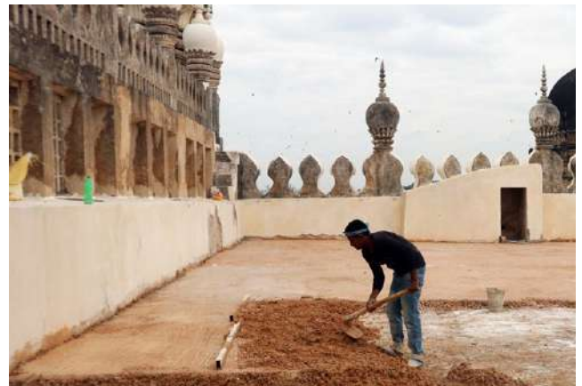
(Above) Dismantling of 20th century cement concrete on the middle terrace; (Below) Traditional lime concrete was laid in appropriate slope
