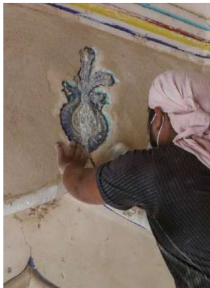
Process of removal of 20th century paint layers from the basalt stone arch crown
