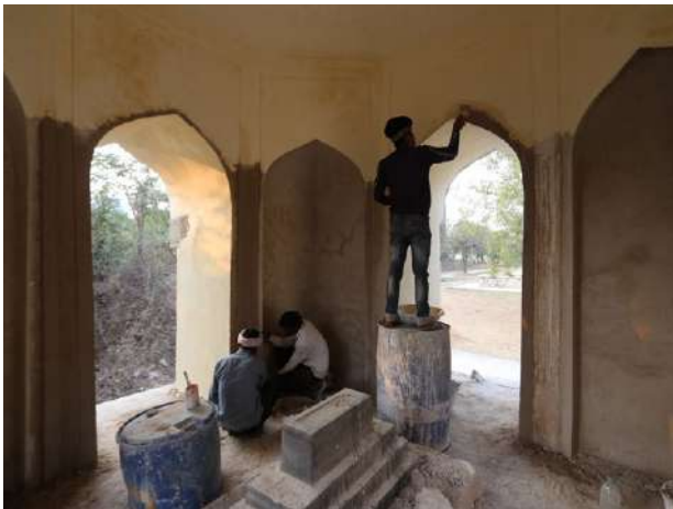
(Left) Plaster repairs were carried out at the internal surface of the tomb; (Right) Missing details on the facade were restored based on in-situ evidence
