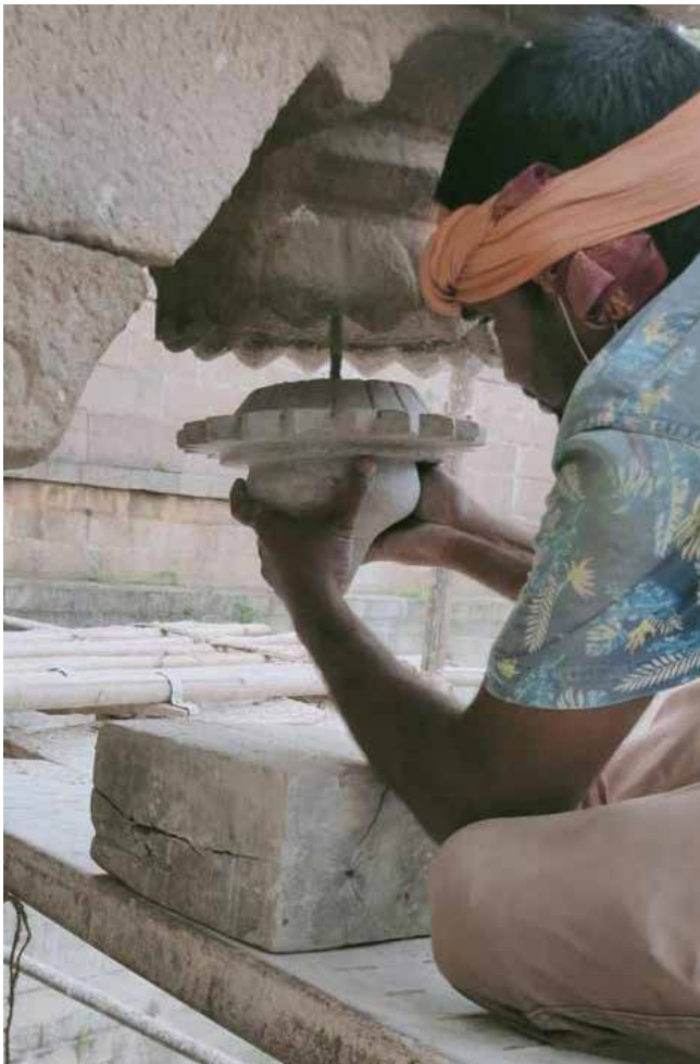
(Left) Installation of bell-shaped motif based on in-situ evidence; (Right) Restoration of the masonry of the ramp - missing stones were reinstated to match the original masonry
