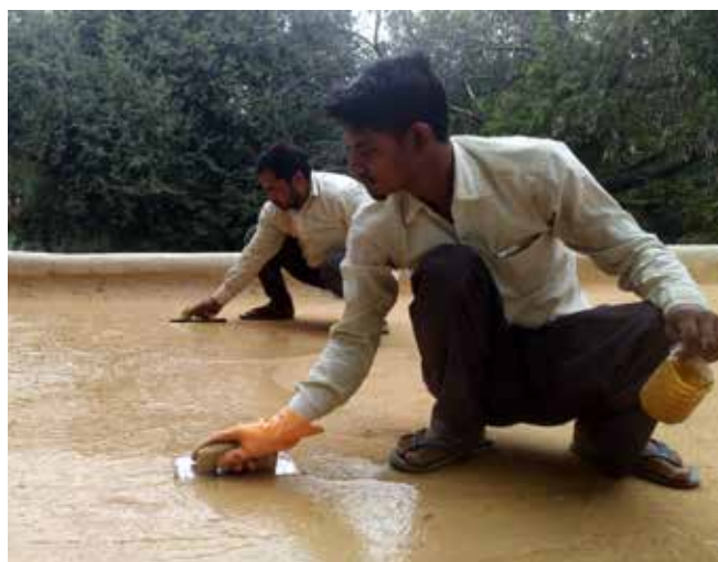
(Left) Spreading and Levelling waterproofing layer on the terrace of Samakhana using traditional aggregates
