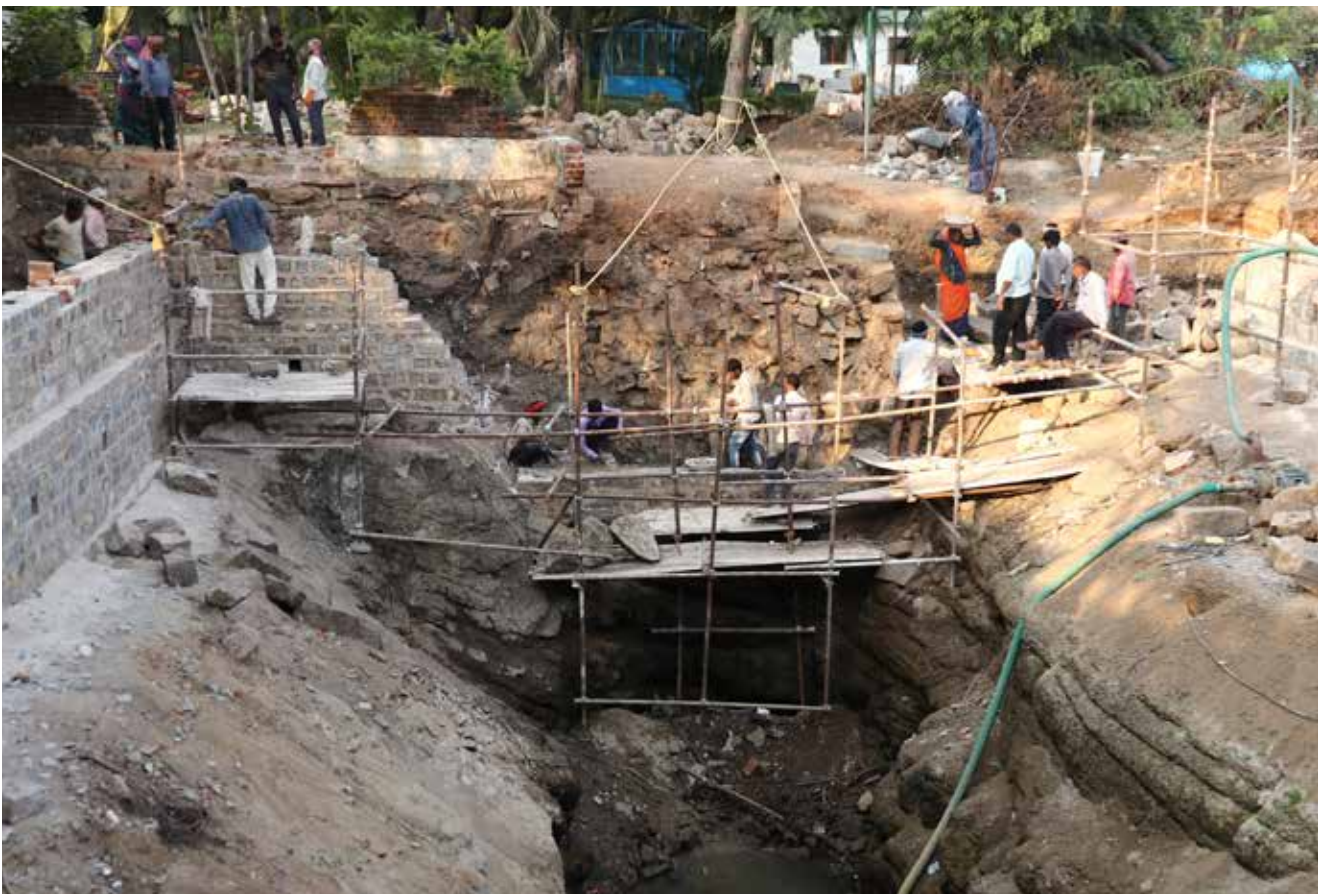
Stone masons restoring the projection in the northern wall as per site-evidence
