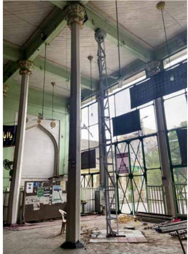
Temporary steel supports installed to support the sagging wooden beam and prevent further displacement on the damaged wooden bracket
