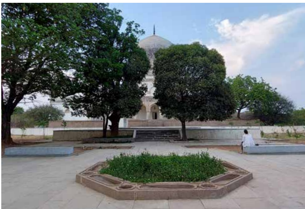
A plaza was developed south of Hayat Bakshi Begum. Brick and stone masonry were removed from the existing fountain, and the dressed stone feature was installed at the finished floor level of the plaza.
