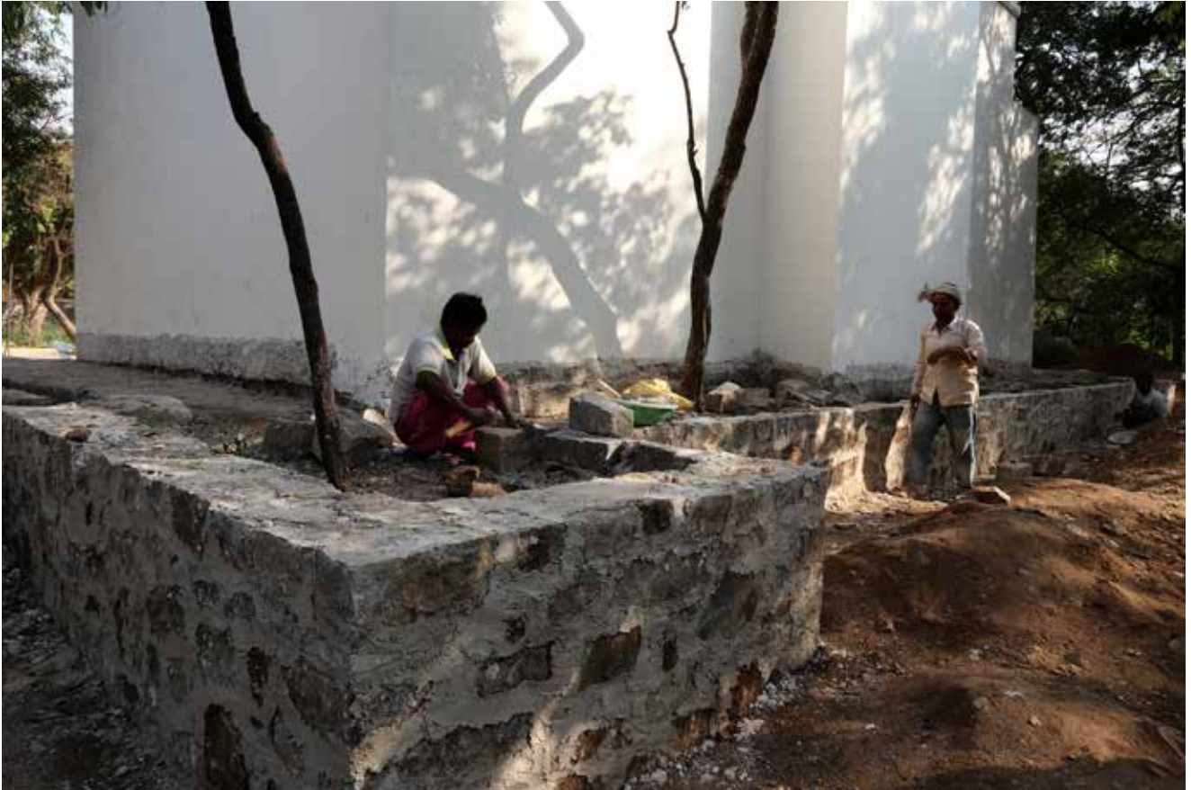
Stone craftsmen installed a plinth protection around the funerary mosque
