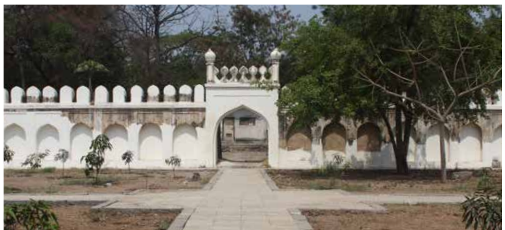
(Top) Battlements on top of the enclosure wall were revealed to the north of funerary mosque of Hayat Bakshi Begum on removal of 20th century cement plaster (Right) Portion of the enclosure wall
