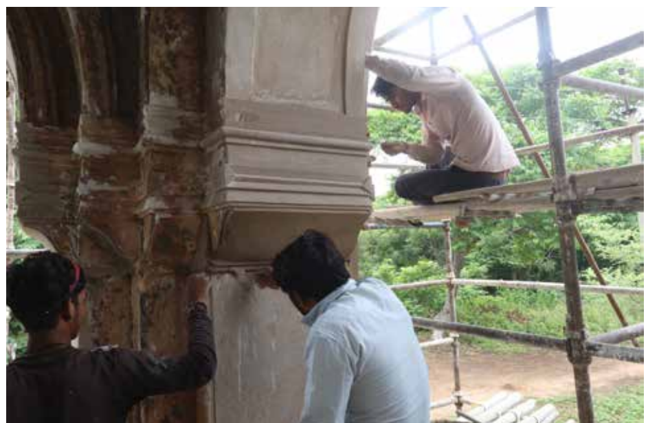
(Above) Ornamental medallion on the internal dome ceiling being restored based on original evidence; (Below) Skilled craftspeople restoring damaged capital bands
