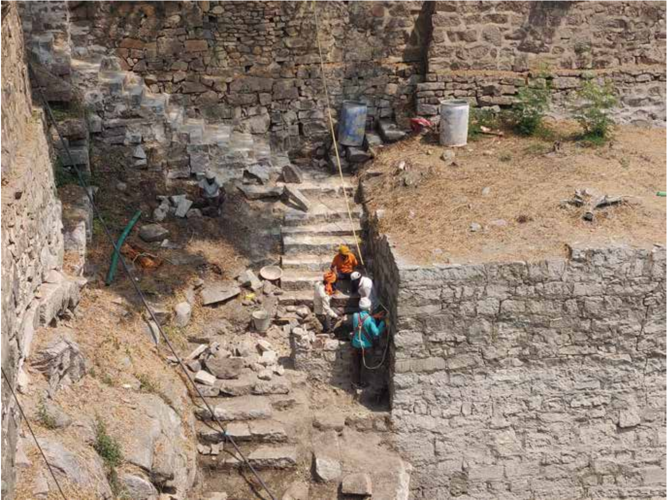
(Above) Installation of missing stone steps
