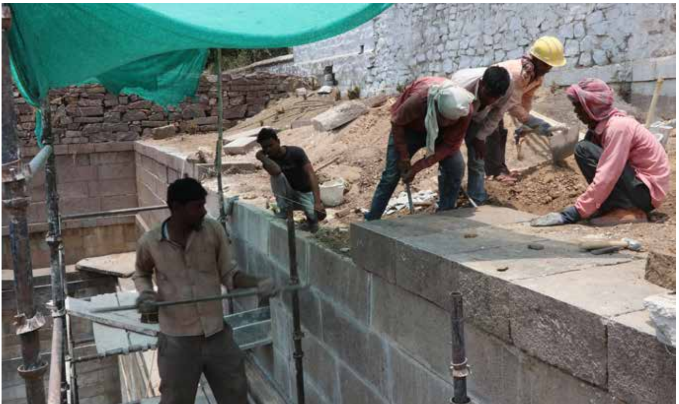
All the displaced dressed stones were reset into place using the existing stones as reference
