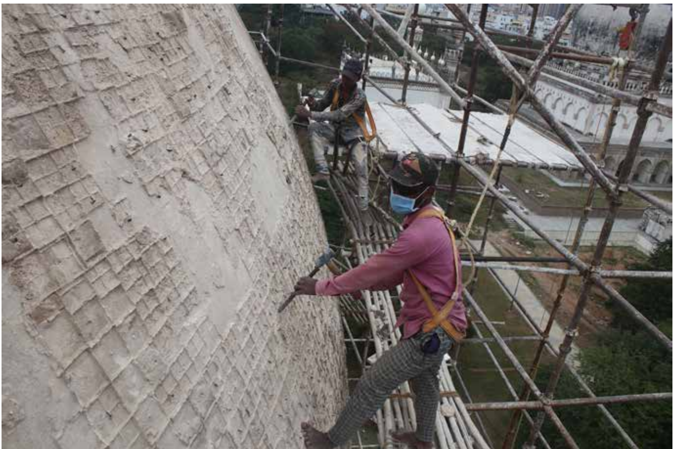
Careful removal of 20 th century cement plaster from the dome revealed historic tiles underneath
