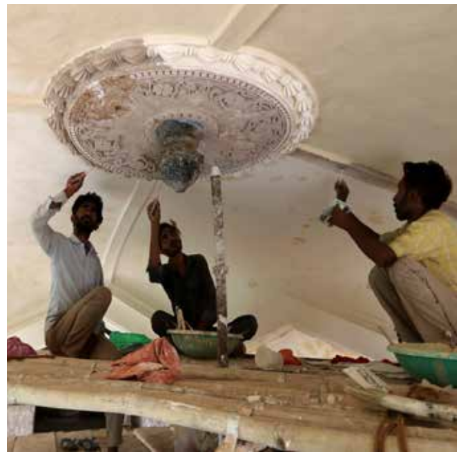
The medallion was restored based on in-situ evidence. A 1:1 scale drawing was prepared to match the existing evidence
