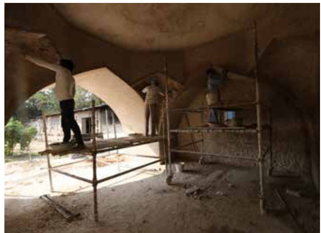
(Left) Stone mason relaying traditional lime concrete on the terrace; (Right) Internal wall surfaces were replastered after dismantling damaged 20 th century cement.
