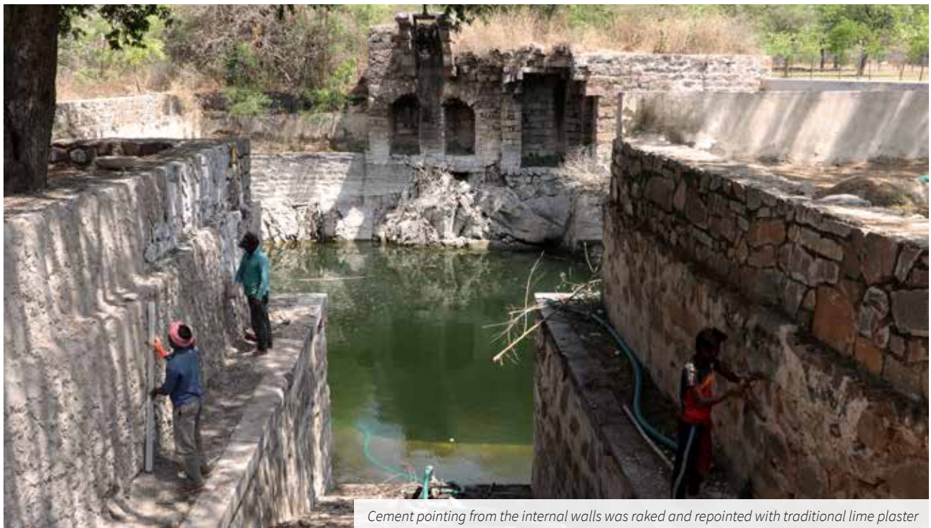
Repointing of the tripartite arch structure with lime mortar
