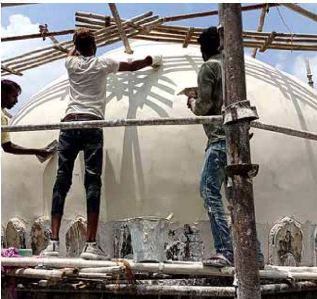
(Left) Final lime punning of the dome after replastering; (Right) Damaged merlons and the decorative bands below them were restored
