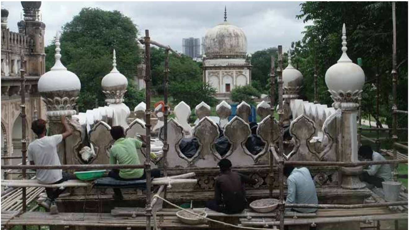
Damaged minarets, missing merlons, and decorative lime stucco details on the parapet being restored carefully by skilled craftsmen
