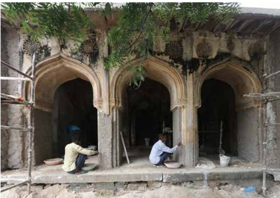
Plaster repairs were carried out on the damaged portions of the internal and external surface of the funerary mosque
