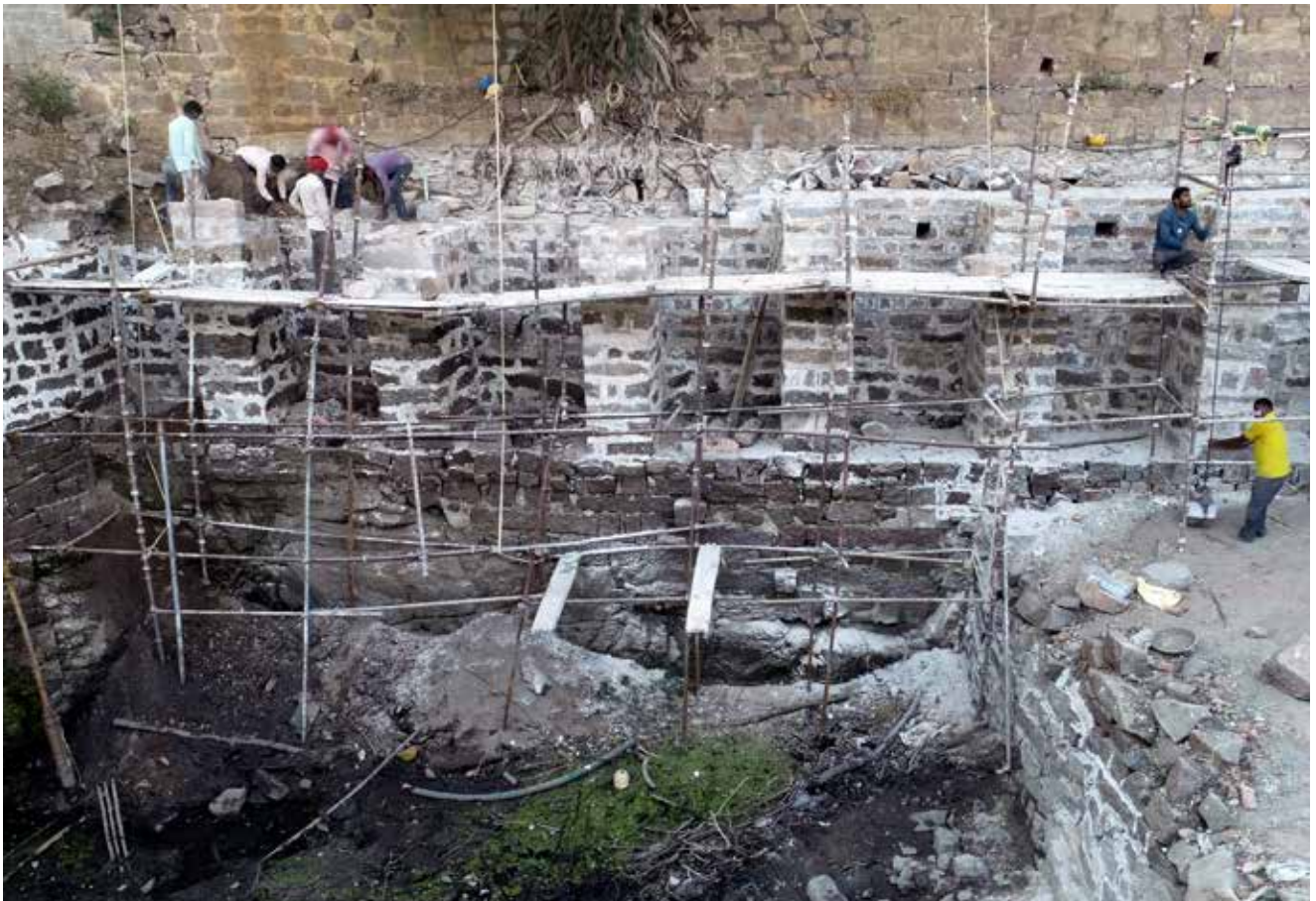
Restoration of buttresses in ashlar masonry to support western retaining wall
