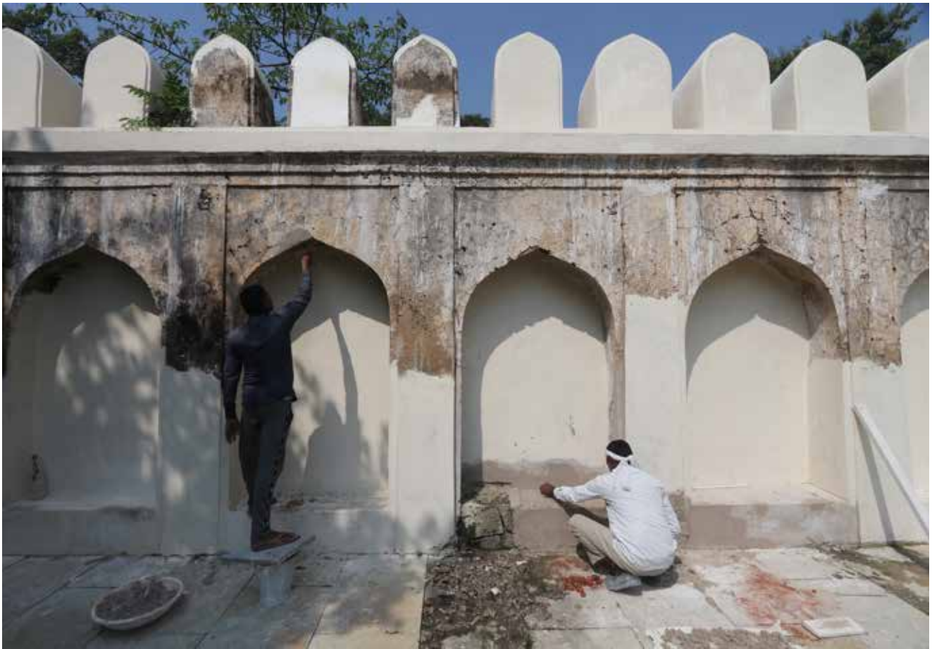
(Top) Damaged portions of the battlements and recessed arches were restored on the south-eastern end of the wall
