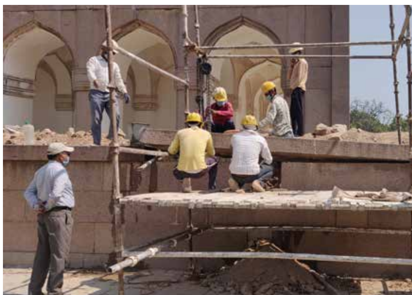
Realignment of the projected plinth by skilled stone masons
