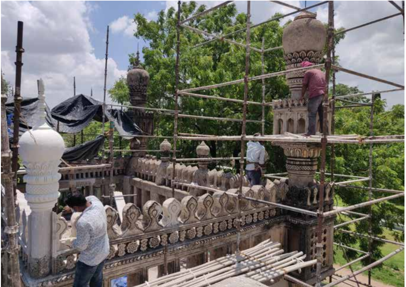
Minarets and the damaged merlons on the parapet walls were reinstated
