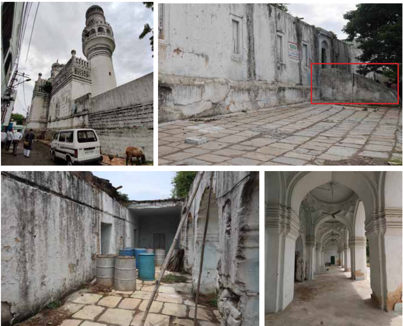
(Clockwise from left) Current principal entrance through a narrow lane; Steps at the original entrance might be demolished due to road widening; Partially collapsed roof of the sarai; Evident signs of water seepage inside the Idgah
