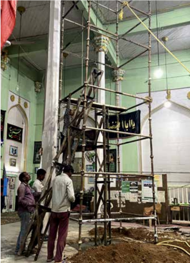
Temporary steel supports installed to support the sagging wooden beam and prevent further displacement on the damaged wooden bracket
