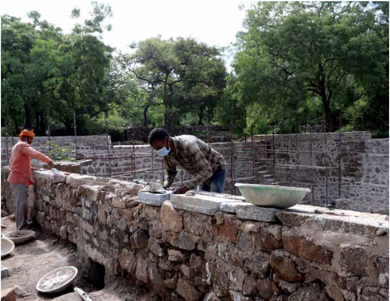
Parapet wall height was raised to ensure visitor safety
