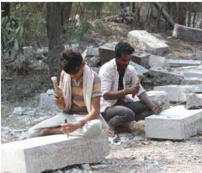
Damaged steps leading into the baoli were replaced with hand-dressed blocks of granite matching the historic evidence
