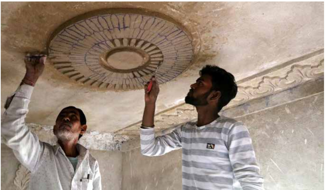
(Clockwise from left) Ornamental stucco band on the ceiling edge restored; Final lime punning layer on the internal walls following the plaster repairs; Ceiling medallion was restored based on original evidence
