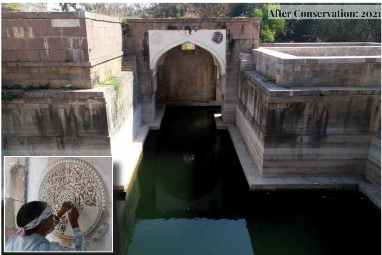
View of the eastern facade of the baoli before and after installation of missing stones, and realignment of displaced stones. The intricate floral medallion was also restored by skilled craftsmen
