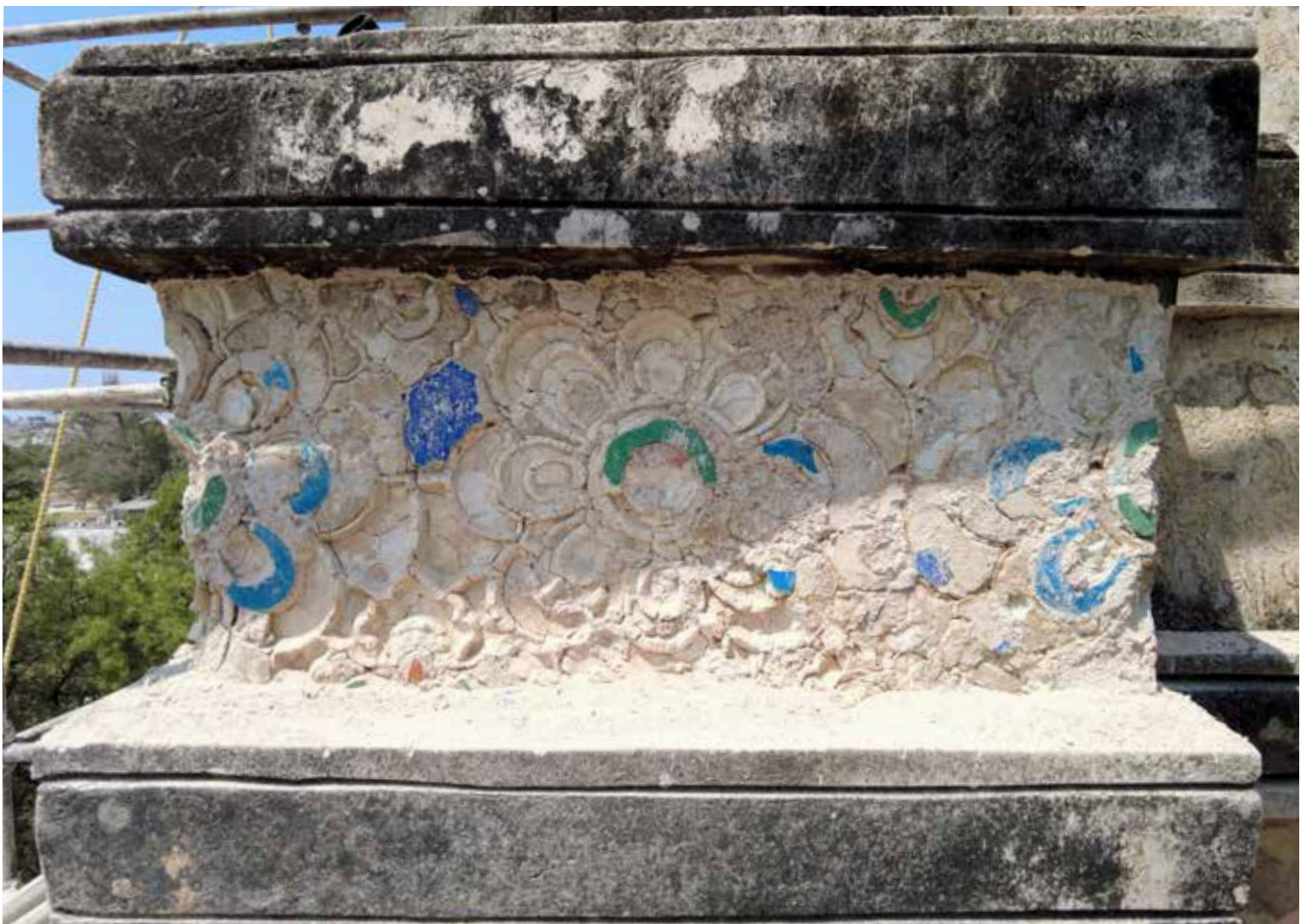
Original lime stucco details with glazed tiles found on removal of 20 th century cement layers from the corner columns
