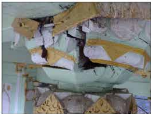
Deteriorating Timber Capital
