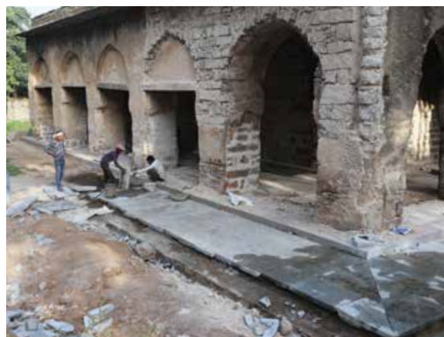
(Left) Removal of cement layer from the interior portions of the monument; (Right) Installation of plinth protection
