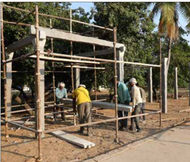
Installation of stone trellises based on vineyard seen in archival images
